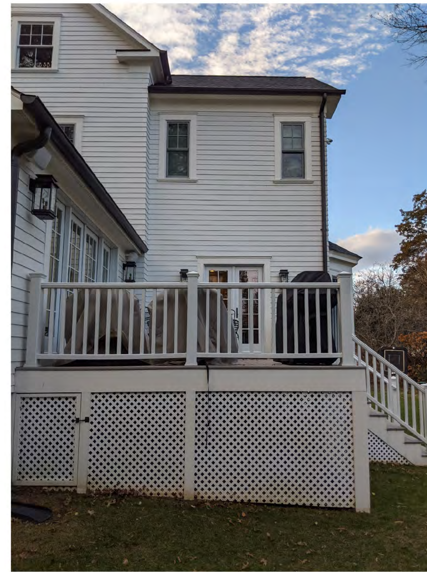
2 11 E. LENOX STREET AREA OF WORK, EAST ELEVATION A702 NOT TO SCALE
