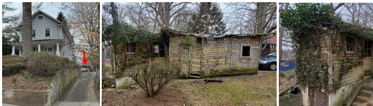
Figure 2: View of the accessory structure from Maple Avenue (left), the south elevation of the accessory structure (center), and the west and south elevations of the accessory structure (right). The red arrow points to the location of the subject structure.
