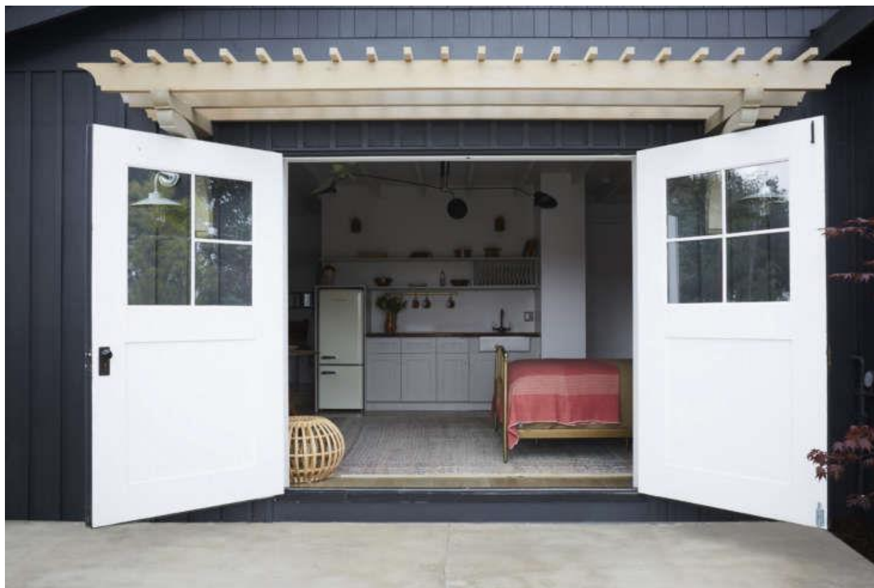
Figure 2: An operable carriage-style door in a converted garage.
