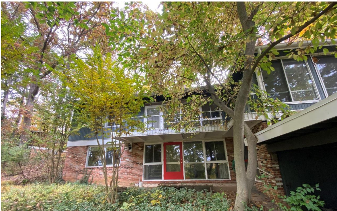
Figure 4: Front elevation of the house showing a full-height window assembly divided into upper (operable)
