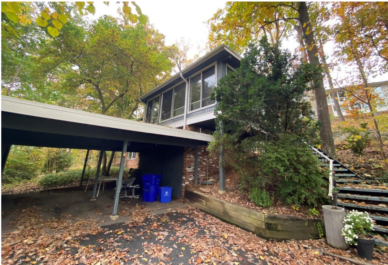
Figure 2: Image showing the existing sunroom window configuration.
