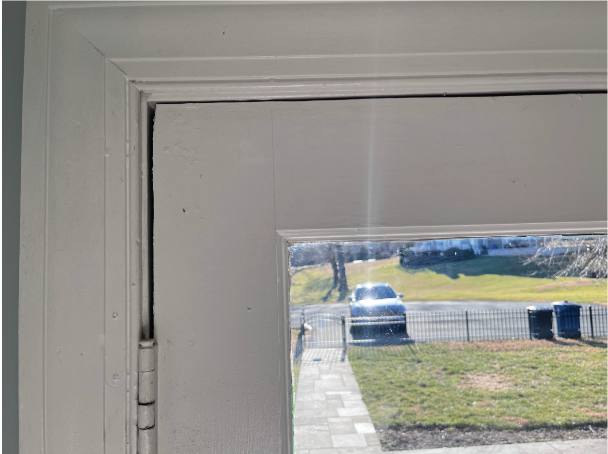
Additional photo showing fit of exterior entryway door in its frame.
