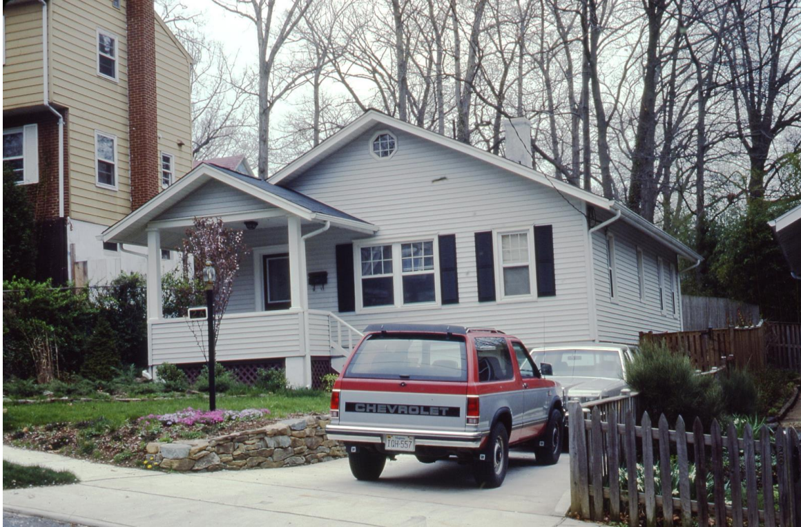
Fig. 2: Subject property prior to 2007 alterations (c. 1980s-90s).
