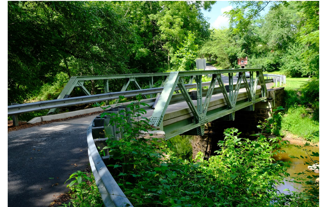
Bridge #M-0030 over Dry Seneca Creek, Montevideo Road (exceptional rustic)
