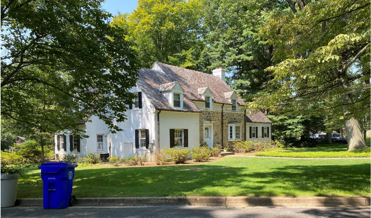
Figure 4: View of 8000 Hampden Lane from the northeast.
