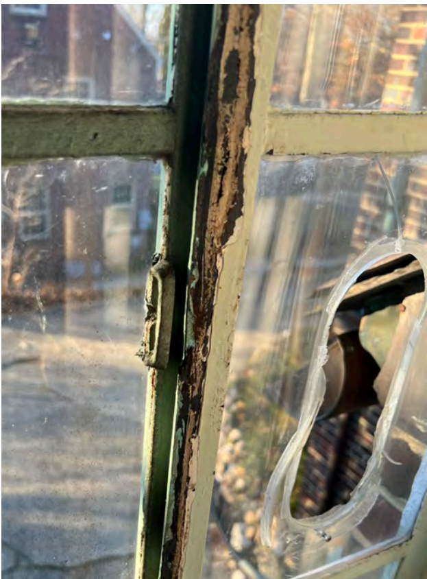
Additional failure of the steel due to rust + missing hardware.
