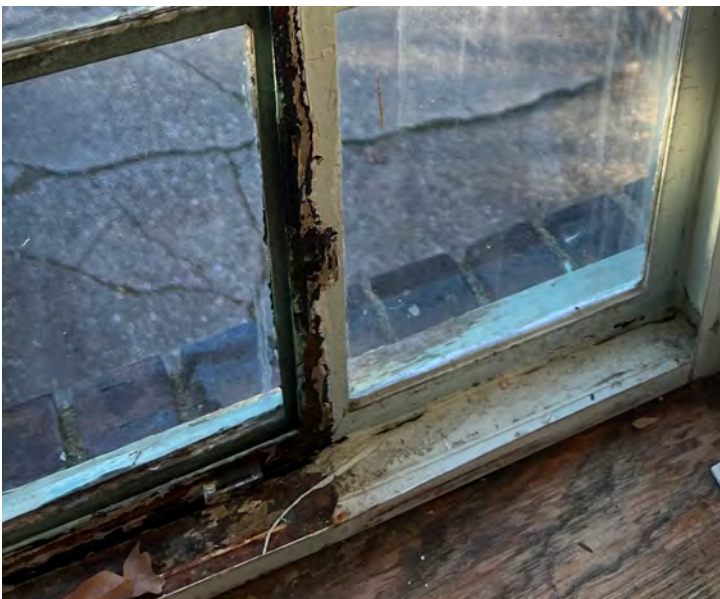
Failure of the steel lower rail due to rust.
