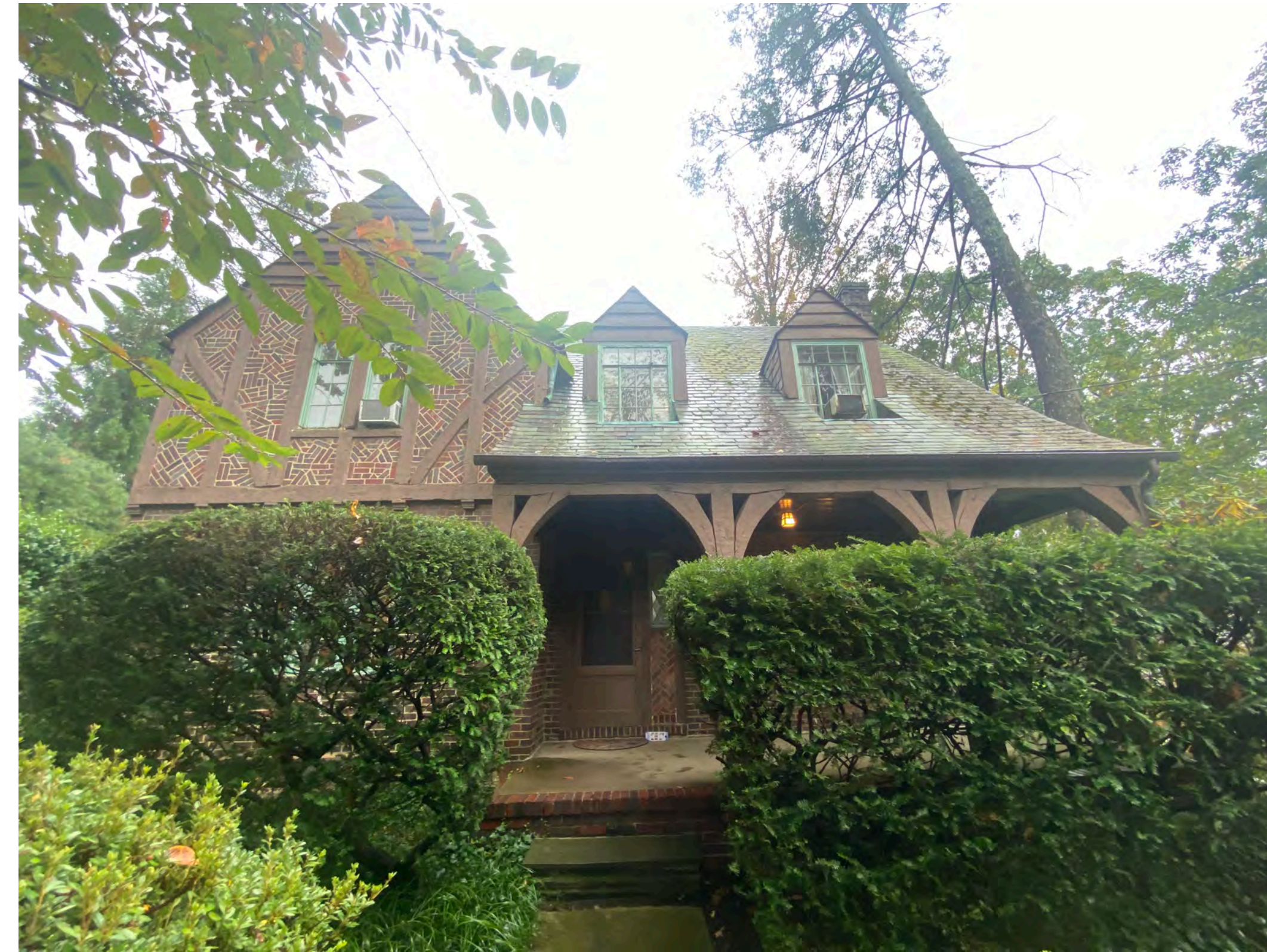
Front north side view
