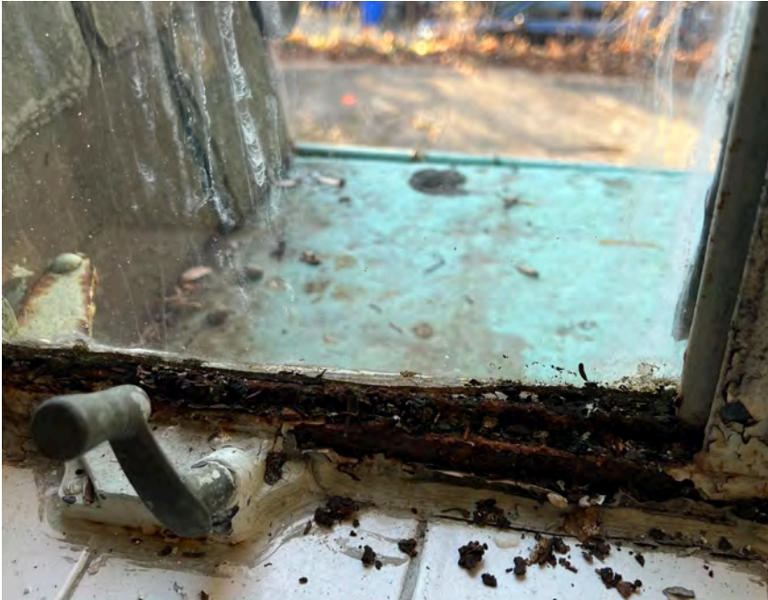
Total failure of the steel lower rail due to rust.
