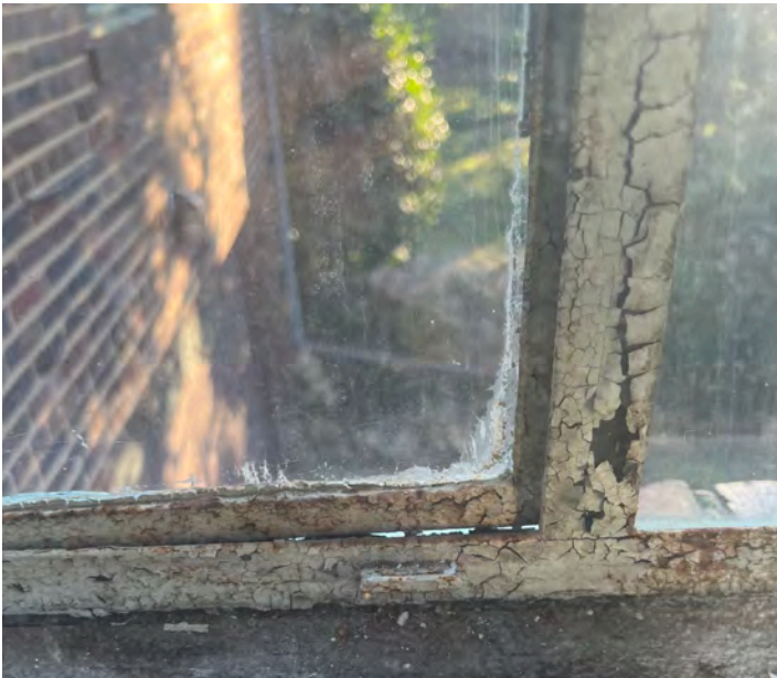
Large gap at the lower edge of a sash
