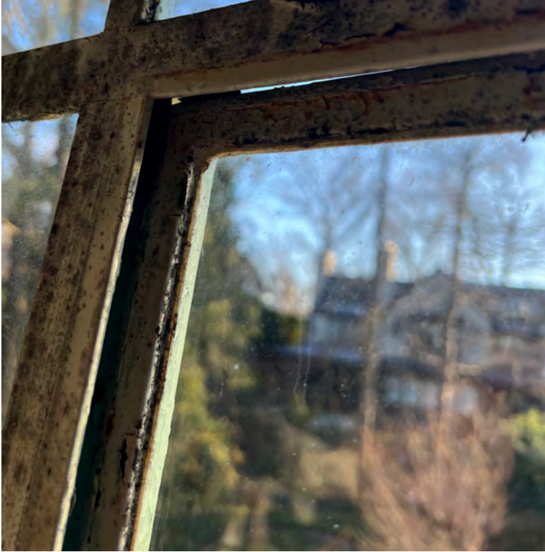
Large gap at the upper edge of a sash
