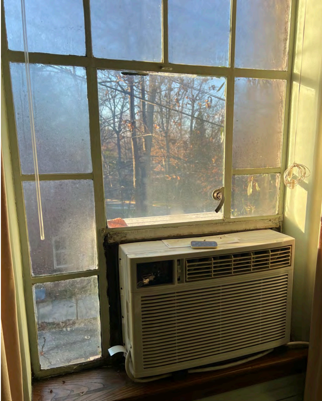
Window cut for installation of AC units (which also caused significant steel damage due to water drainage.)
