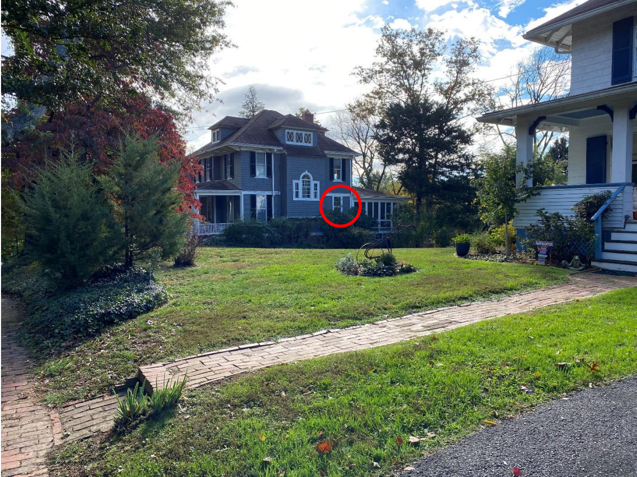
Figure 2: Right elevation of the subject property. The enlarged window opening is circled in red.
