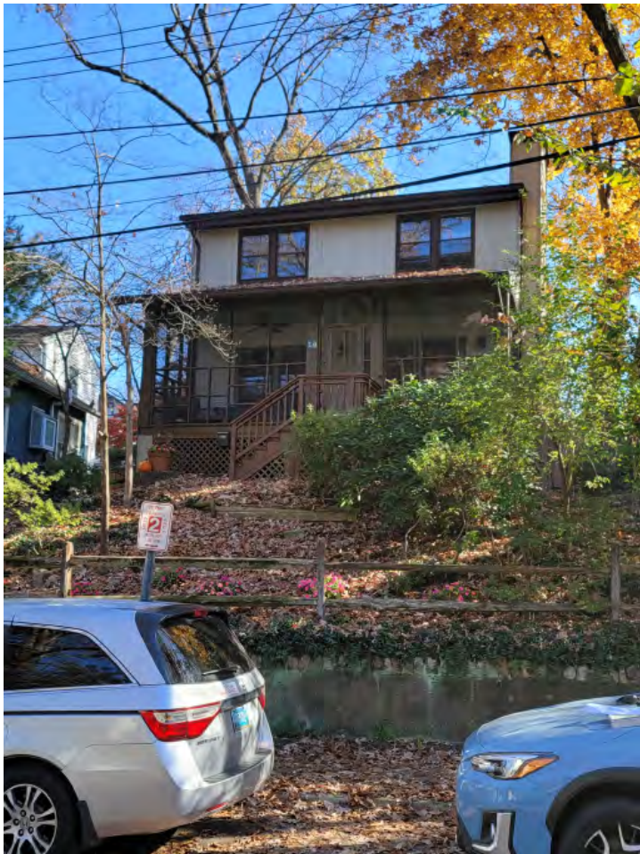
Existing Photo Front Elevation
