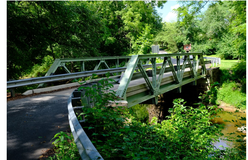
Truss bridge over Dry Seneca Creek on Montevideo Road
