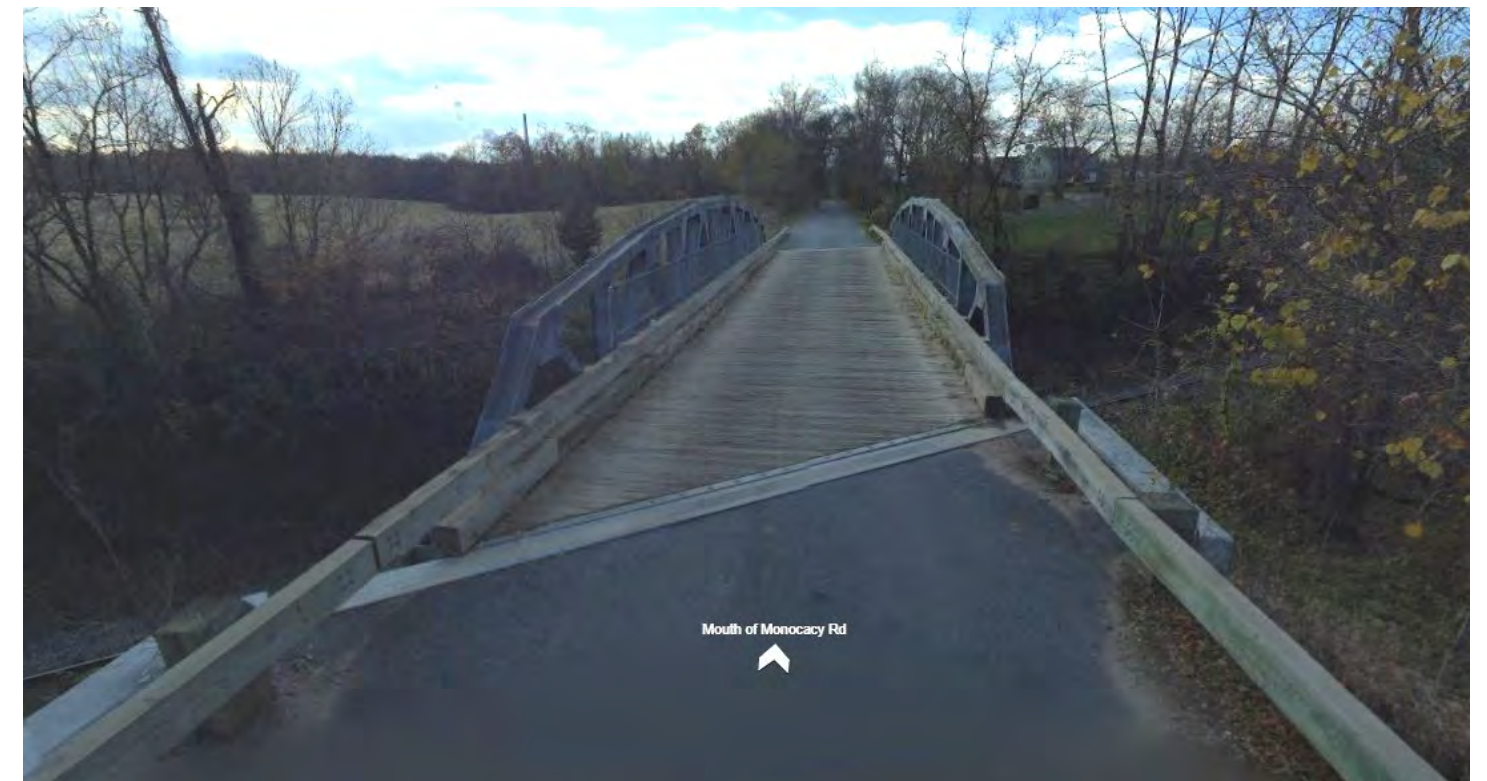
Bing Streetside Image of Bridge #M-0135
