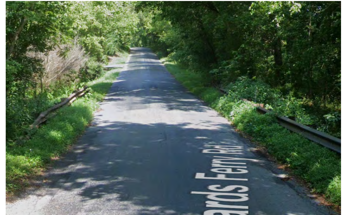
Google Street View of Bridge #M-0181
