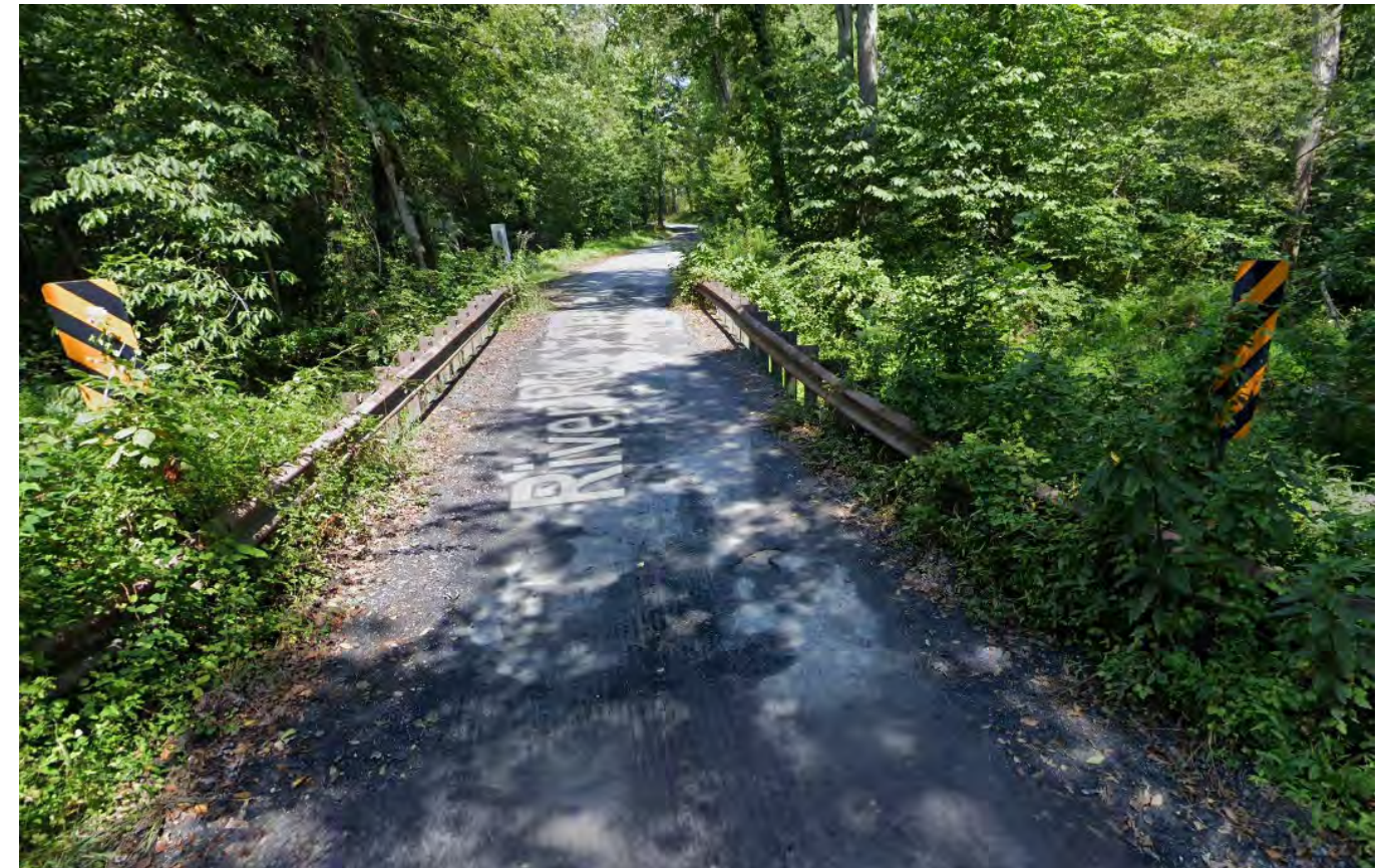
Google Street View of Bridge #M-0040
