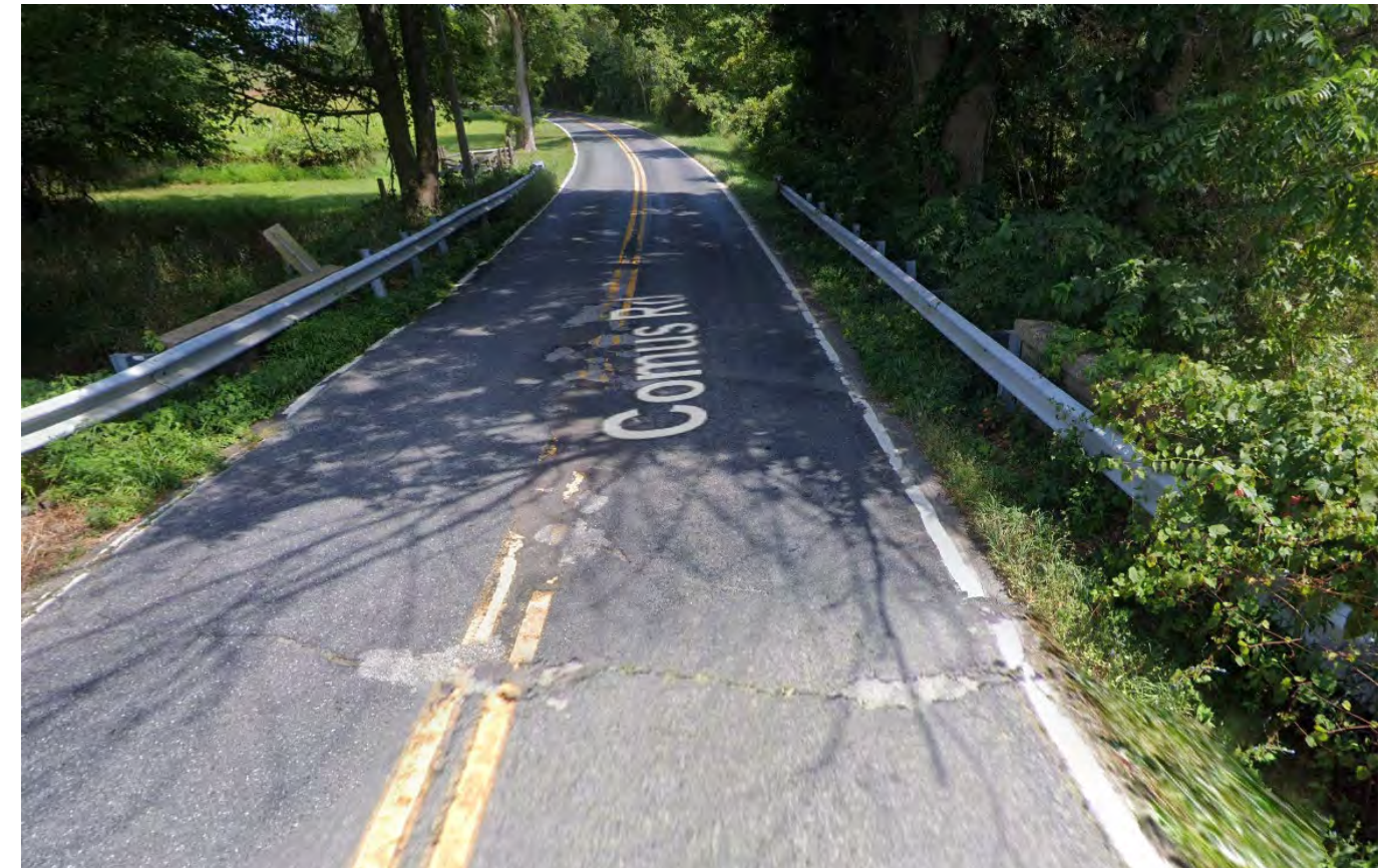
Google Street View of Bridge #M-0296
