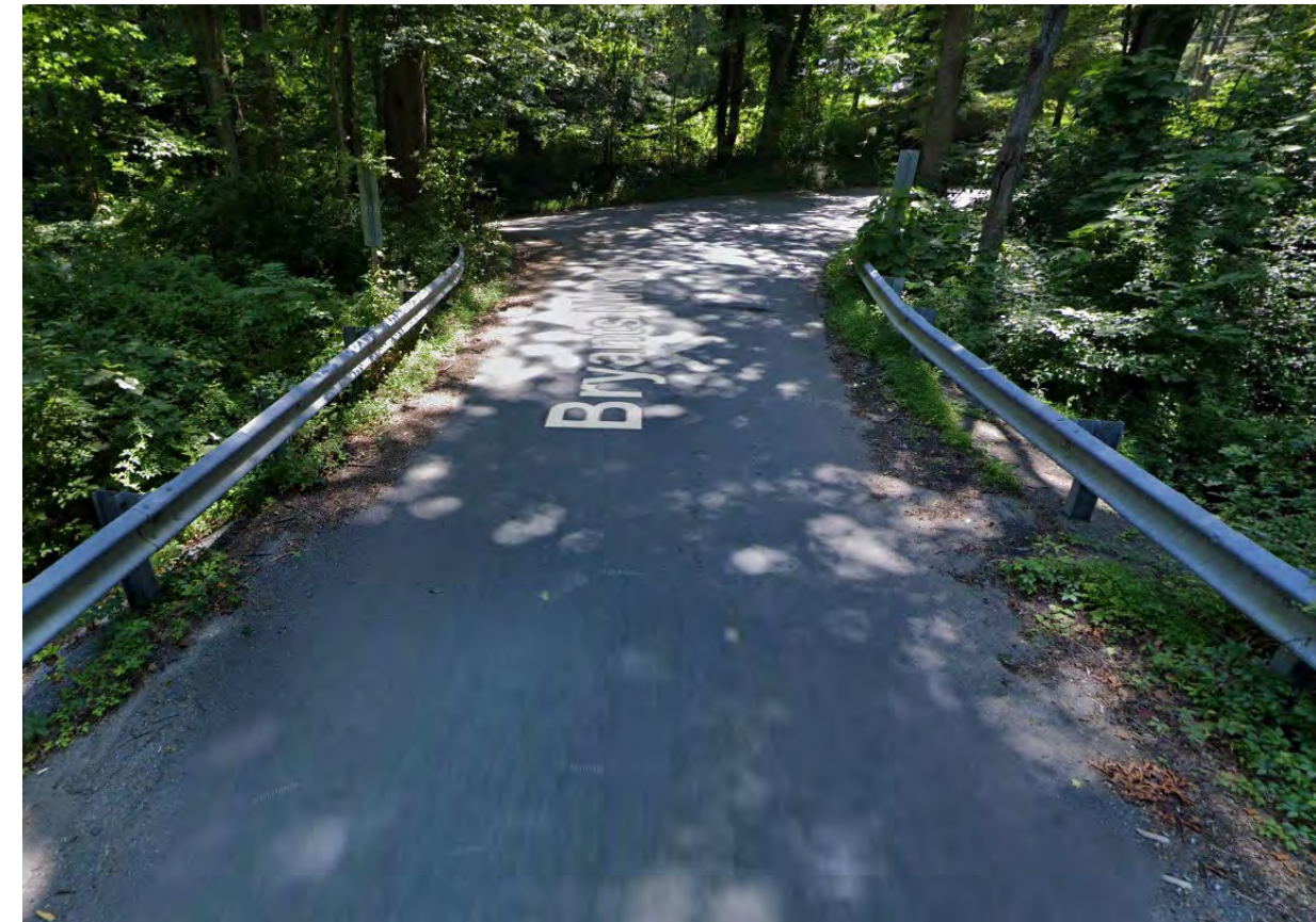
Google Street View of Bridge #M-0313
