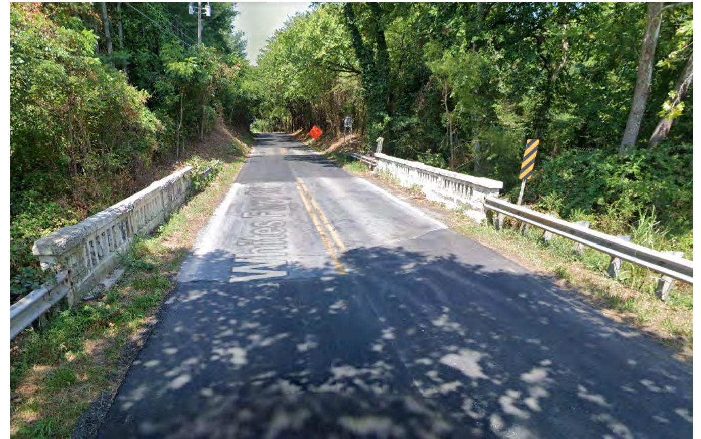
Google Street View of Bridge #M-0186
