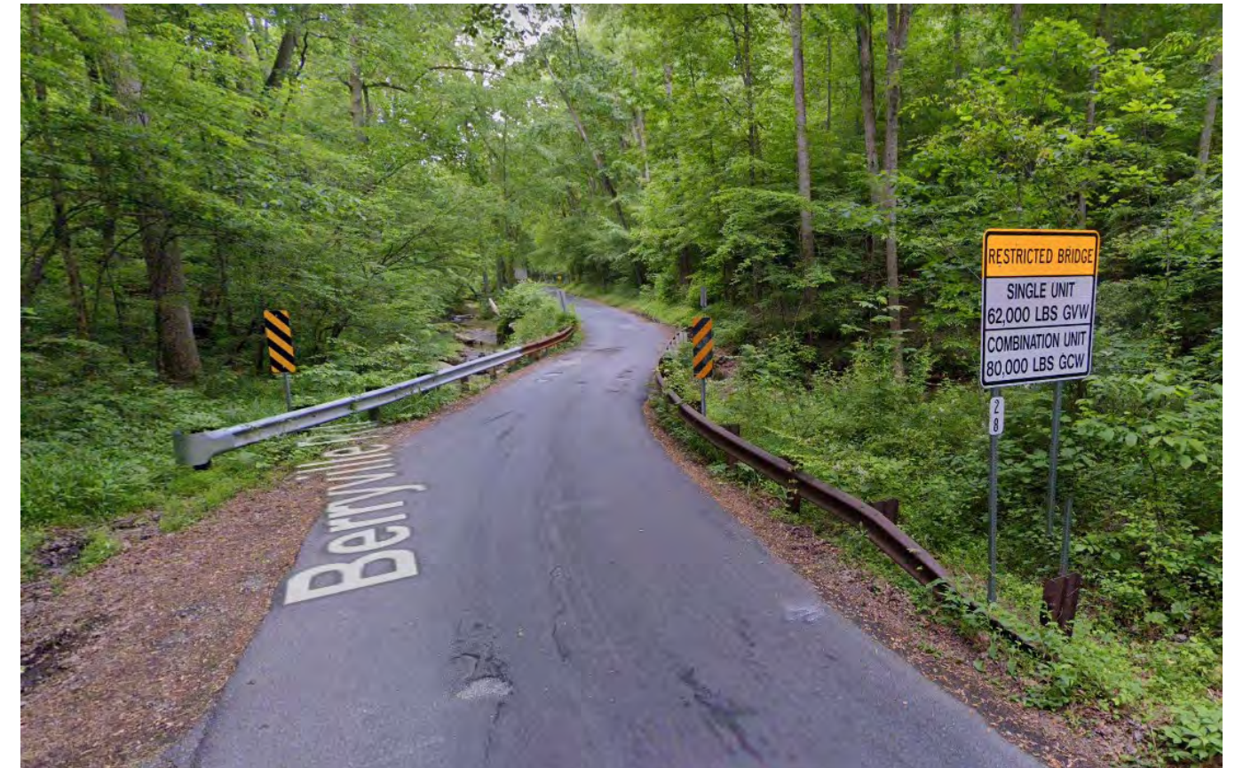
Google Street View of Bridge #M-0028
