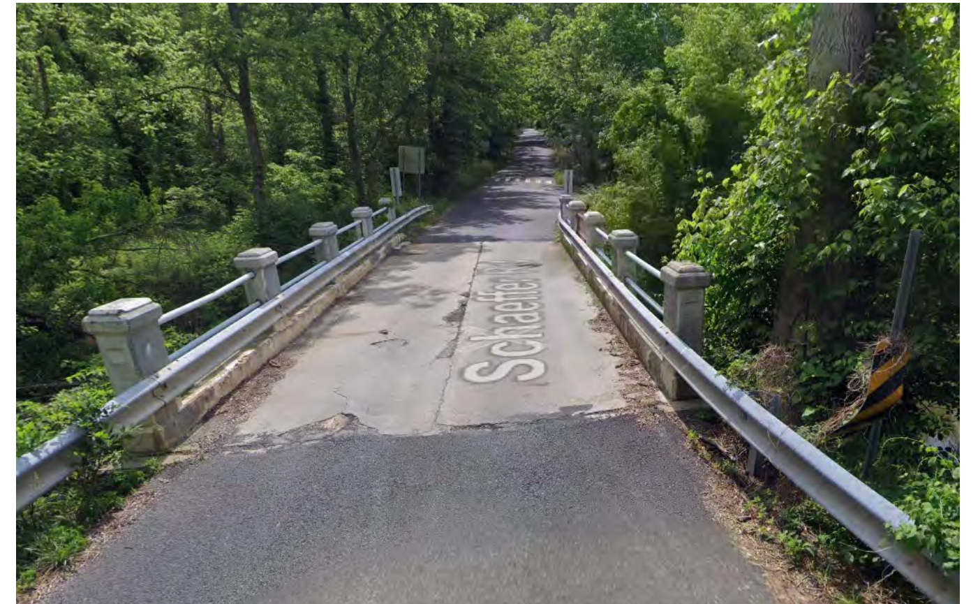
Google Street View of Bridge #M-0137
