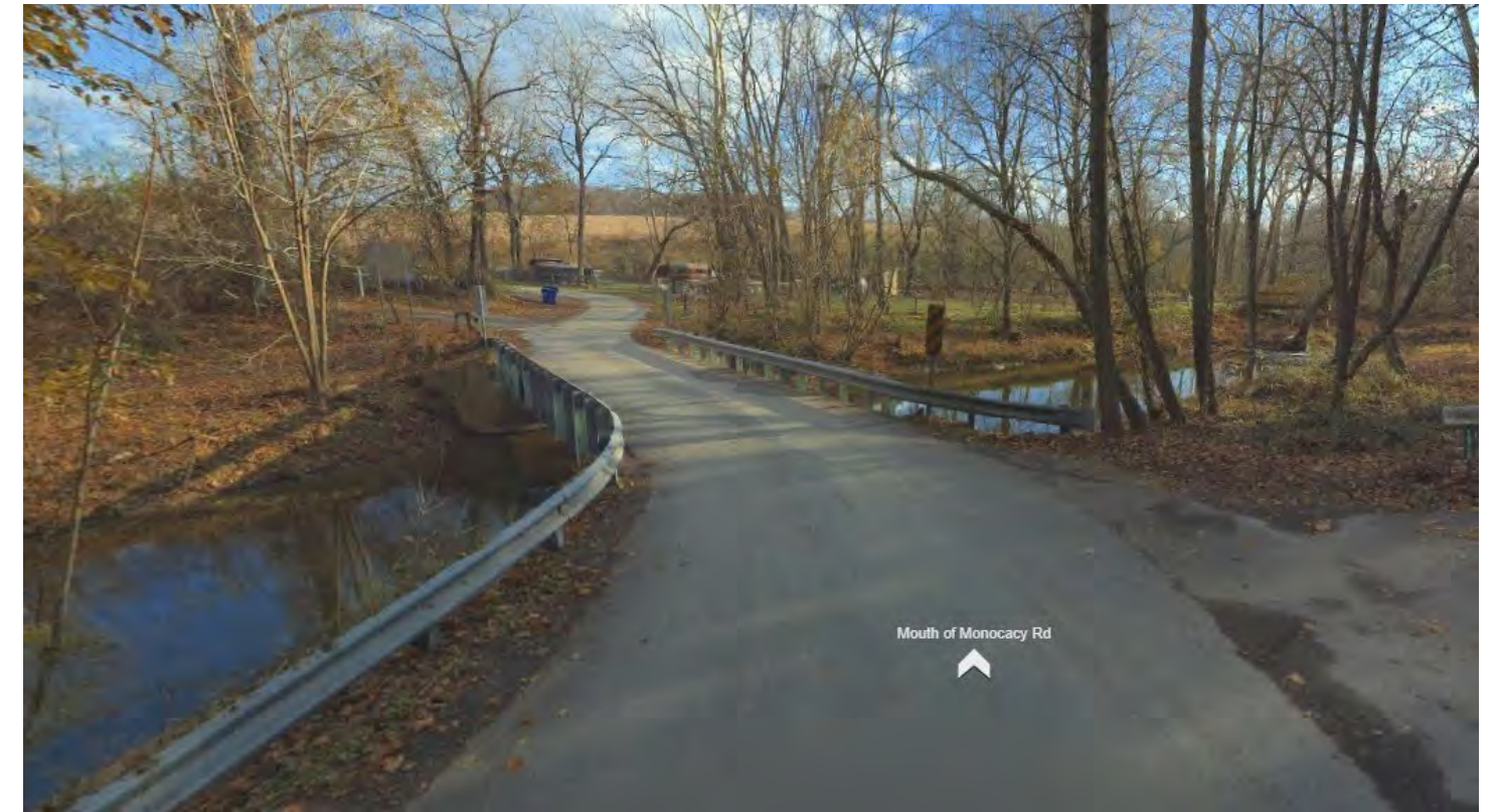
Bing Streetside Image of Bridge #M-0043
