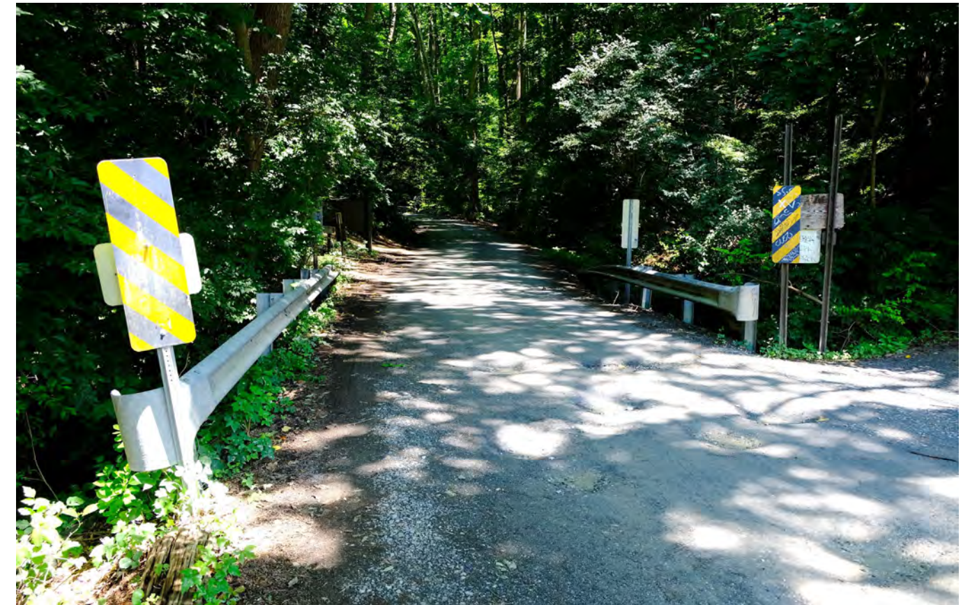
Google Street View of Bridge #M-0022
