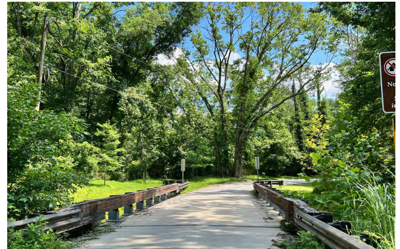
Planning Staff Image of Bridge #M-0030
