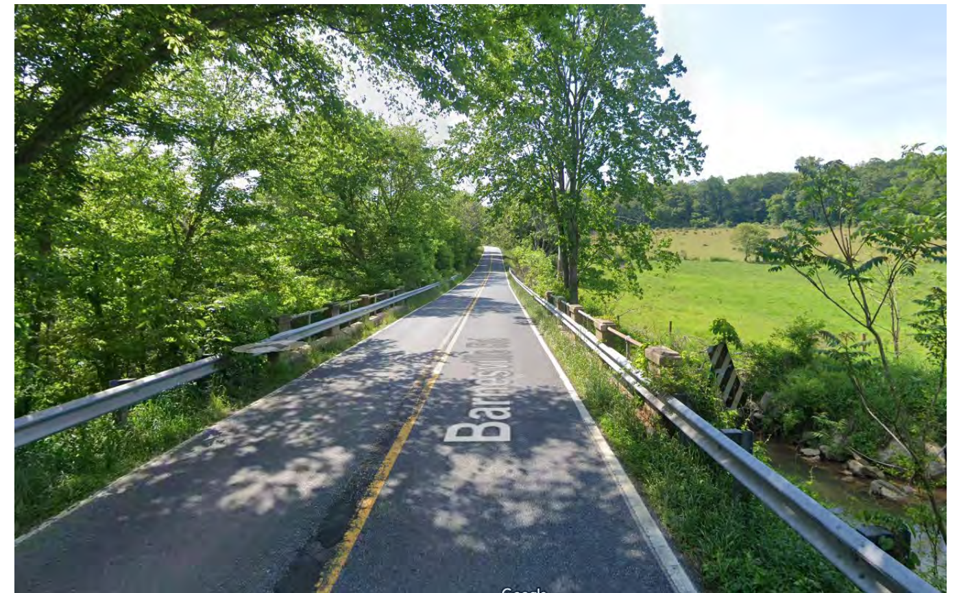
Google Street View of Bridge #M-0045
