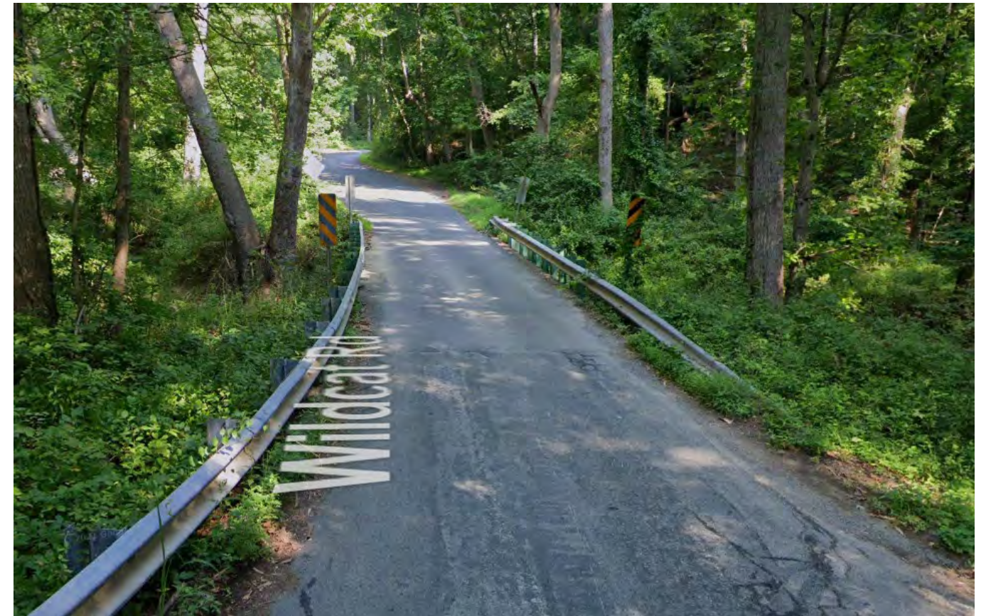
Google Street View of Bridge #M-0068
