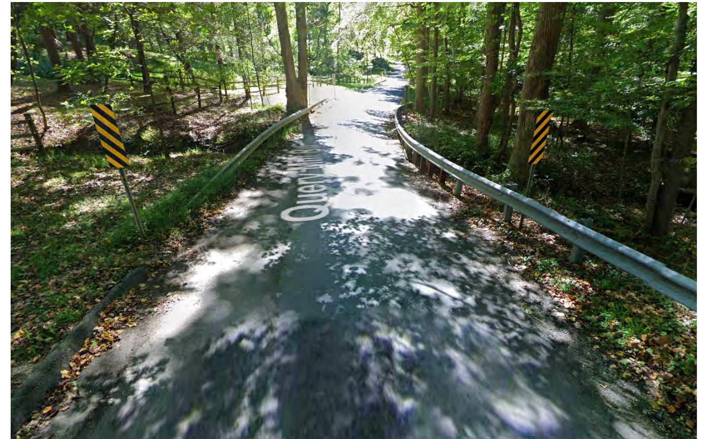
Google Street View of Bridge #M-0020
