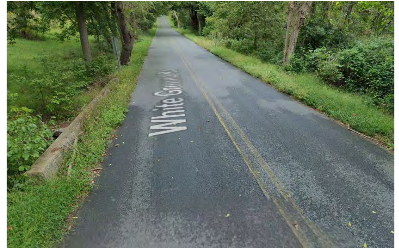
Google Street View of Bridge #M-299
