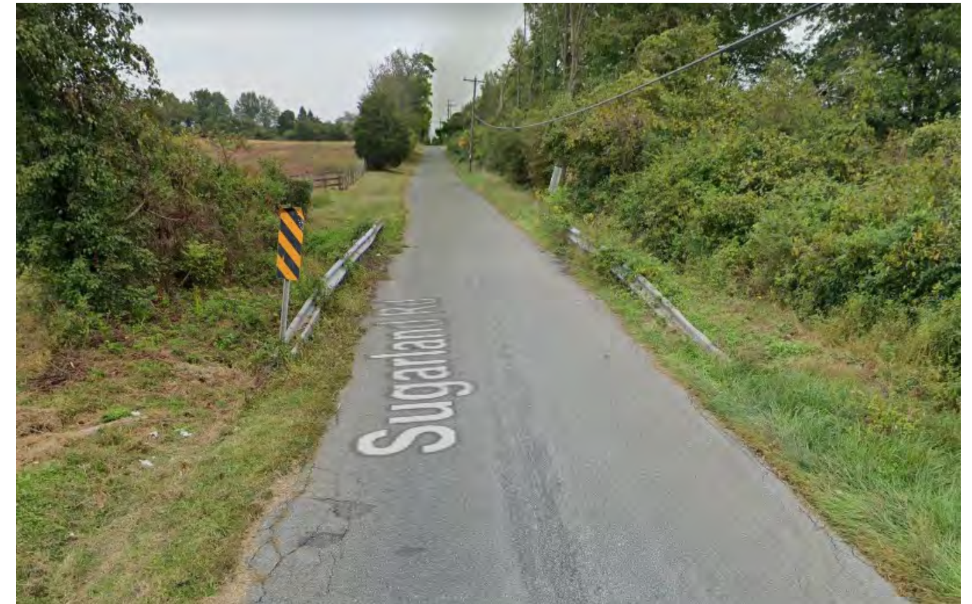
Google Street View of Bridge #M-0034
