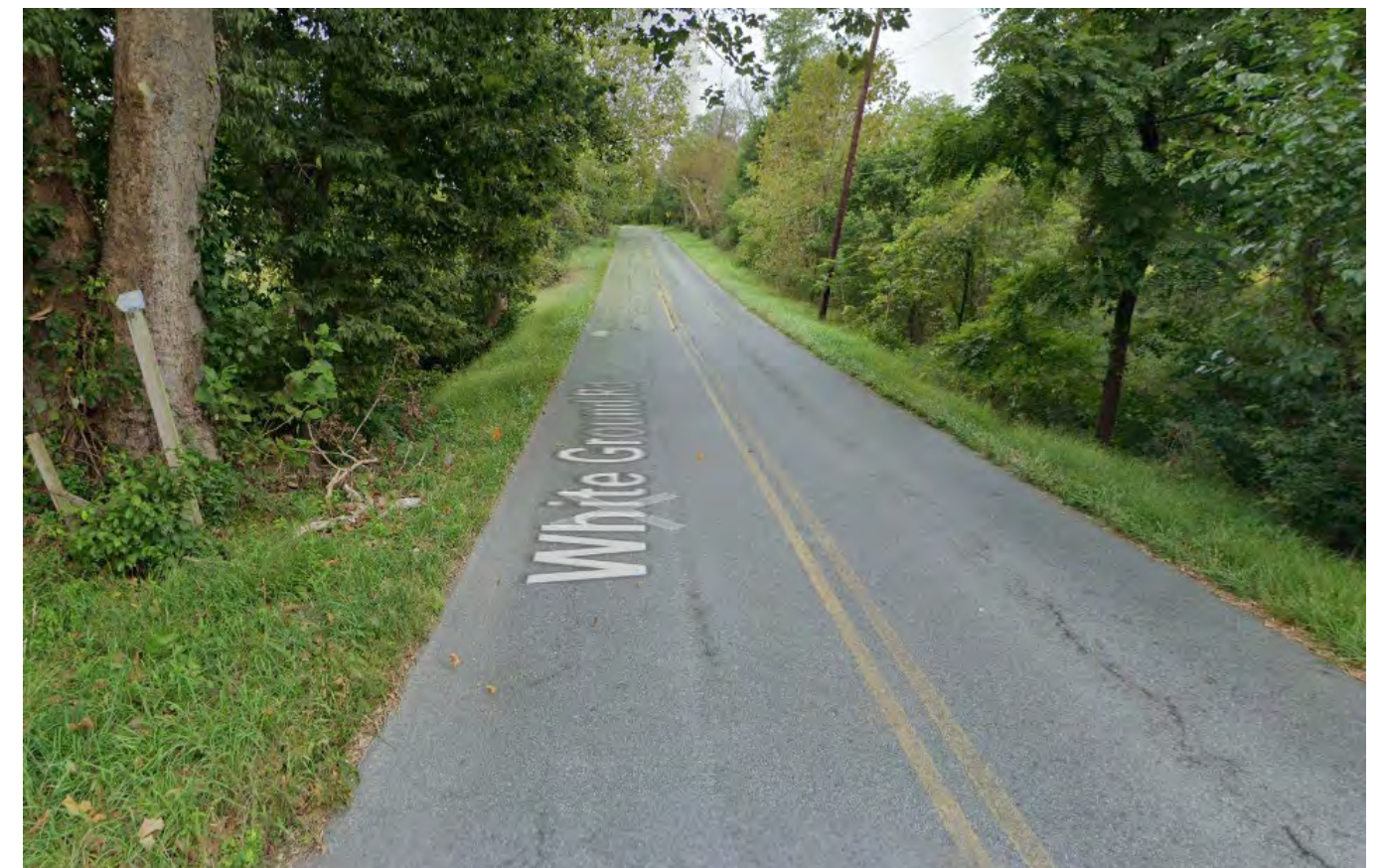
Google Street View of Bridge #M-0300
