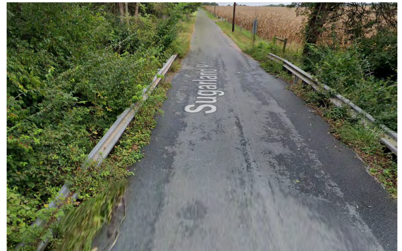
Google Street View of Bridge #M-0035
