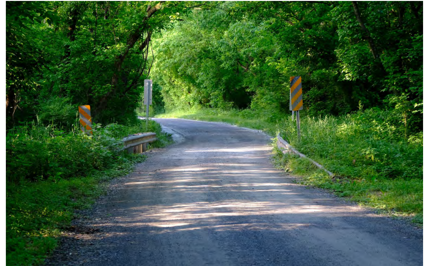
Google Street View of Bridge #M-0031
