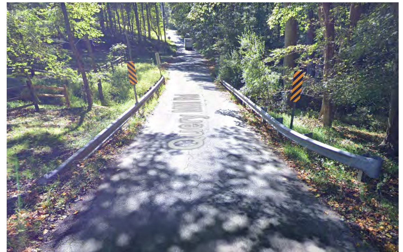
Google Street View of Bridge #M-0329
