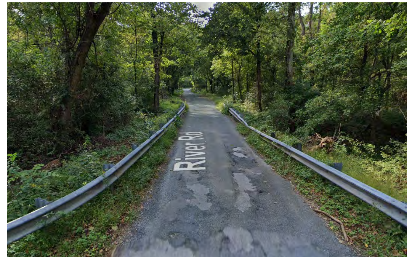
Google Street View of Bridge #M-0039
