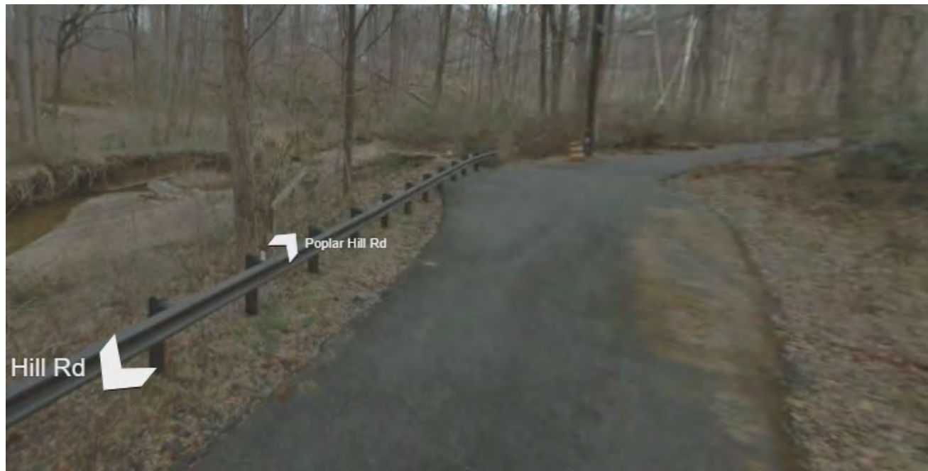
Bing Street View of the end of the southern segment of Poplar Hill Rd
