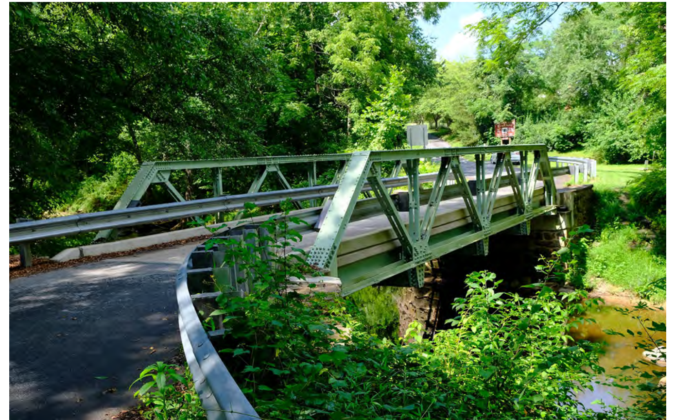
Planning Staff Image of Bridge #M-0030
