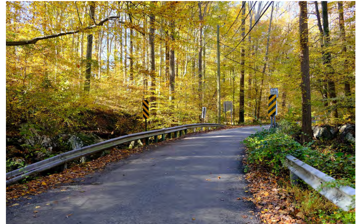
Planning Staff Image of Bridge #M-0019
