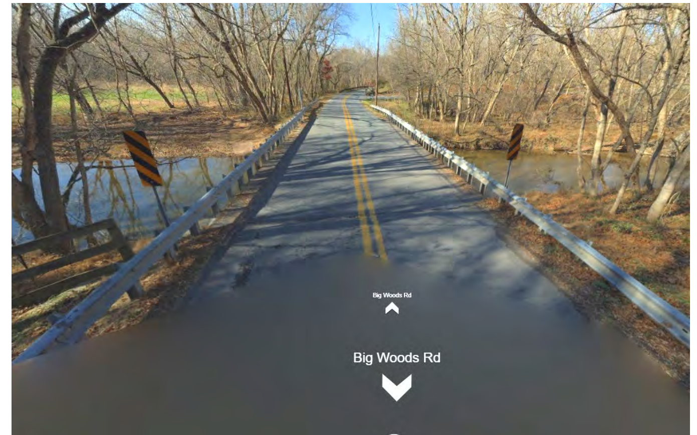
Bing Street View of Bridge #M0044
