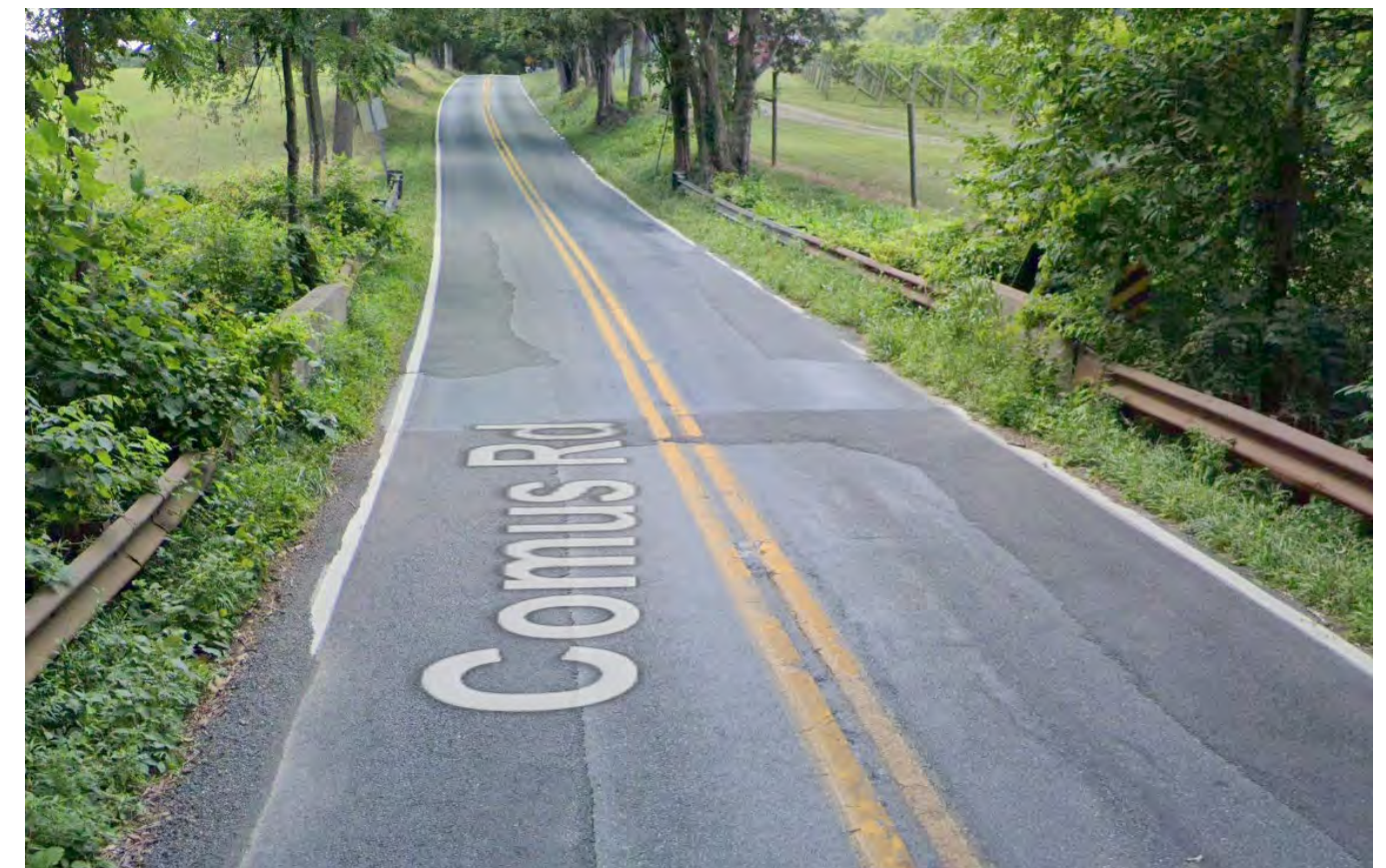
Google Street View of Bridge #M-0302
