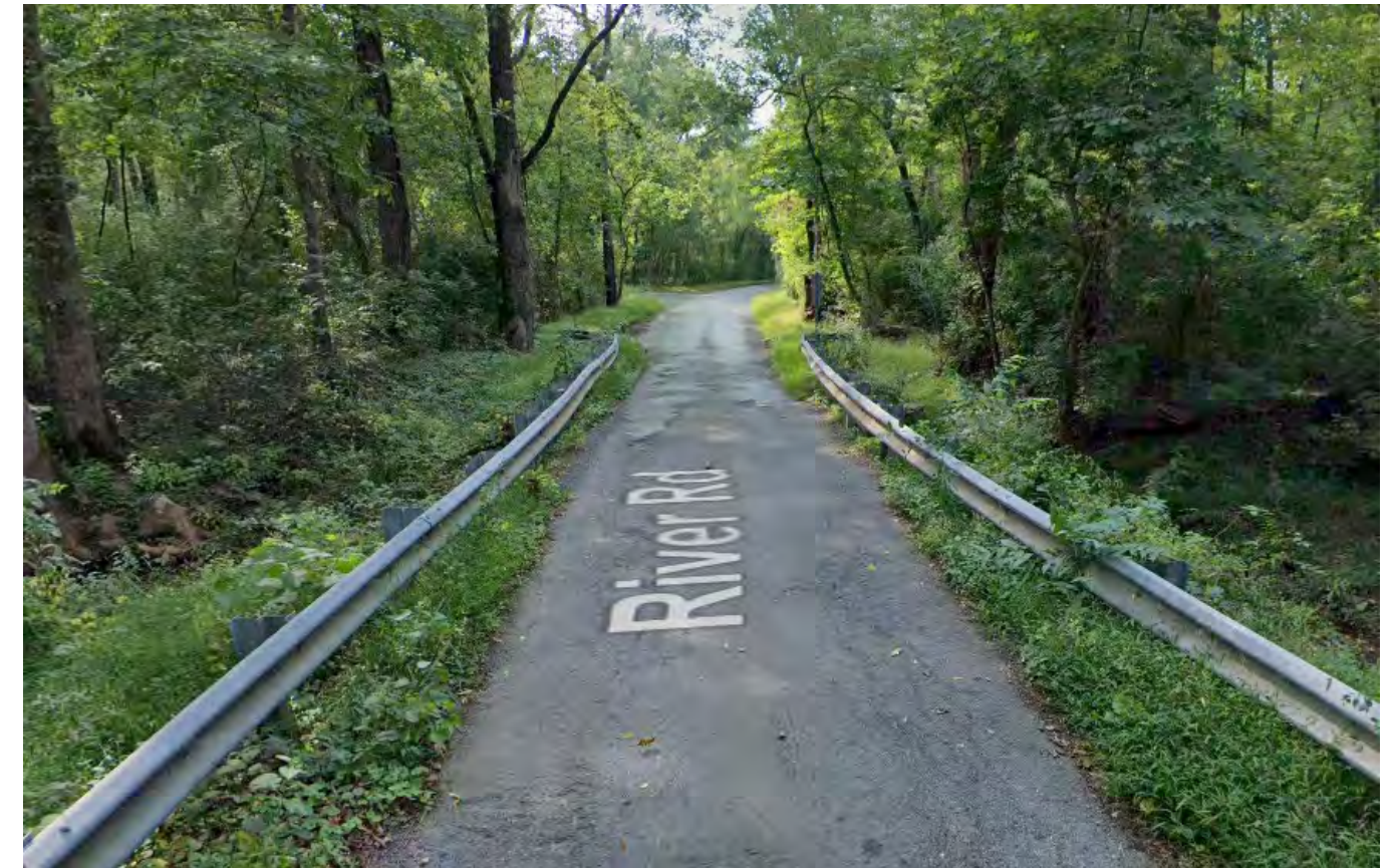
Google Street View of Bridge #M-0038
