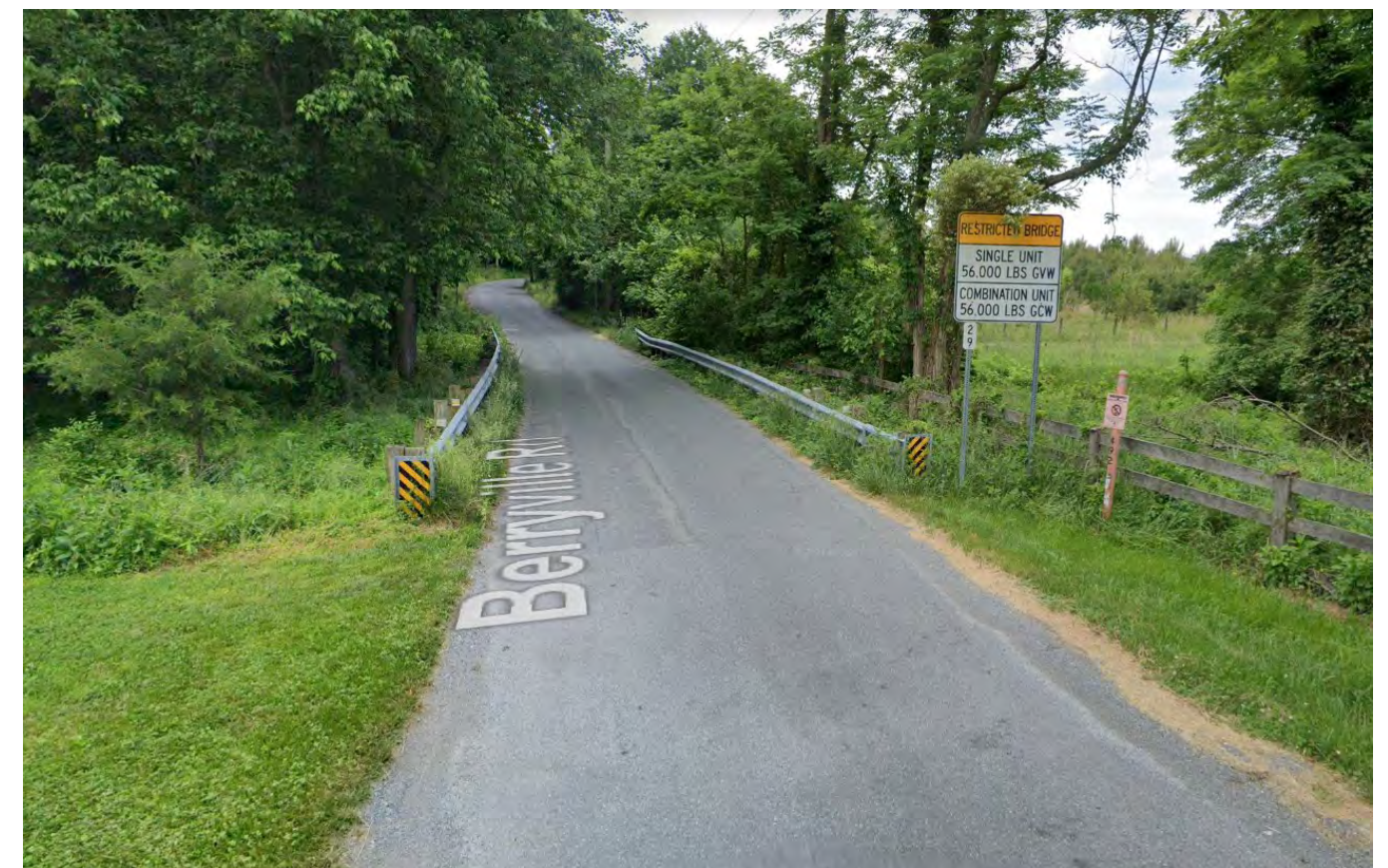
Google Street View of Bridge #M-0029
