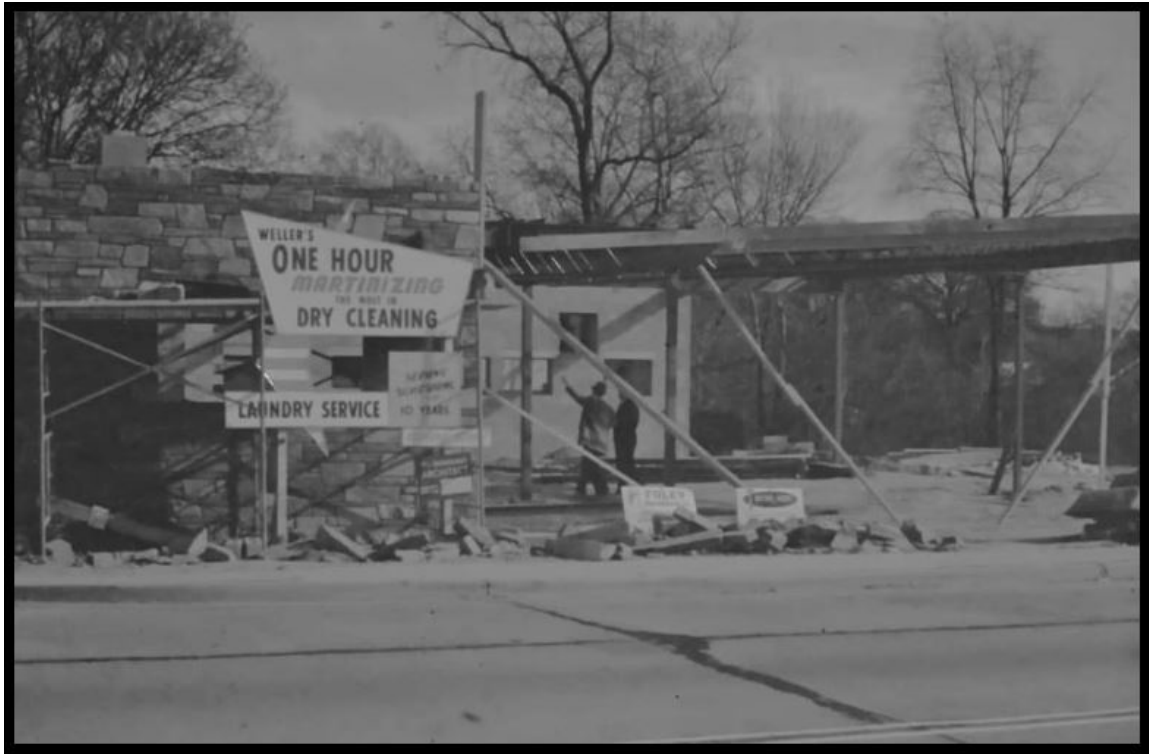
Figure 2: View of the Weller's Dry Cleaning under construction, ca. 1961. Note the sign that reads "Weller's One Hour Martinizing The Most in Dry Cleaning." The framing for the glazed projecting section and the concrete block wall on the rear elevation are visible. Source: Courtesy of Rose Jean Weller/Silver Spring Historical Society.
