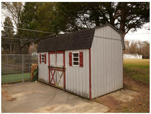
Figure 17: View of a wood-frame, gambrel-roof, shed (Outbuilding G).
