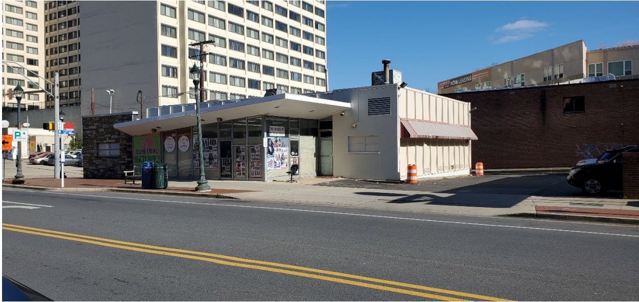
Figure 1: View of the front elevation from across Fenton Street, November 2022.
