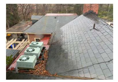
View of existing north flat seam roof with existing mechanical units.
