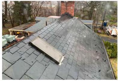
View of existing slate shingle roof with existing skylight.
