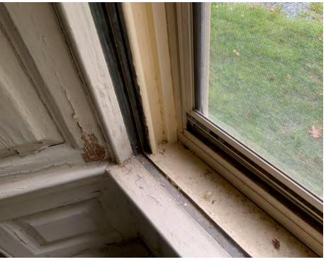
Aluminum sash track in historic windows of foursquare, interior side of exterior aluminum frame storm window visible.
