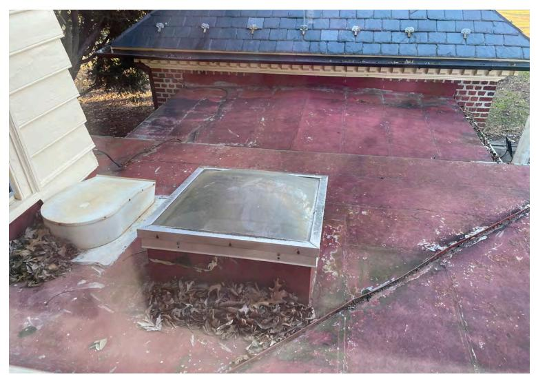
View of existing north flat seam roof with existing vent and skylight.
