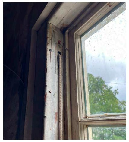
Sash pulley and counterweight rope exists in many window located, however some are broken or missing.
