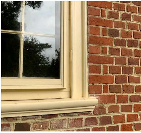
Evidence of prior shutter hinge see in patched area of exterior window trim. Surrounding masonry has been re-pointed in several locations concealing former shutter dog anchoring devices.
