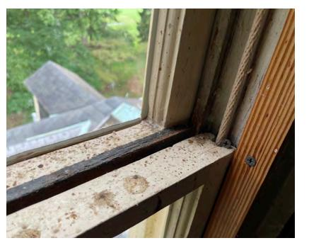
Select windows have been secured shut using screws in jambs.
