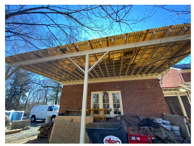
Existing maintenance storage area along north wall of garage, covered by shed roof structure.
