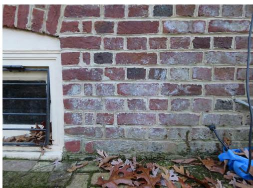
Efflorescence Cleaning Tests – Cathedral Stone Efflorescence Remover was the most successful cleaner but did not remove all the efflorescence (red box).
