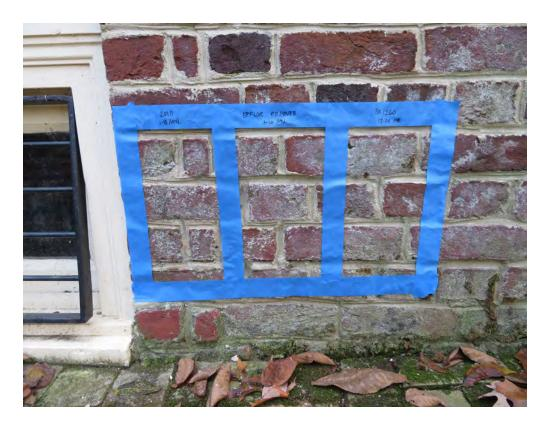
Efflorescence Cleaning Tests (left to right) – Prosoco 2010 All Surface Cleaner, Cathedral Stone Efflorescence Remover, and Prosoco 1260 Limestone & Marble Poultice
