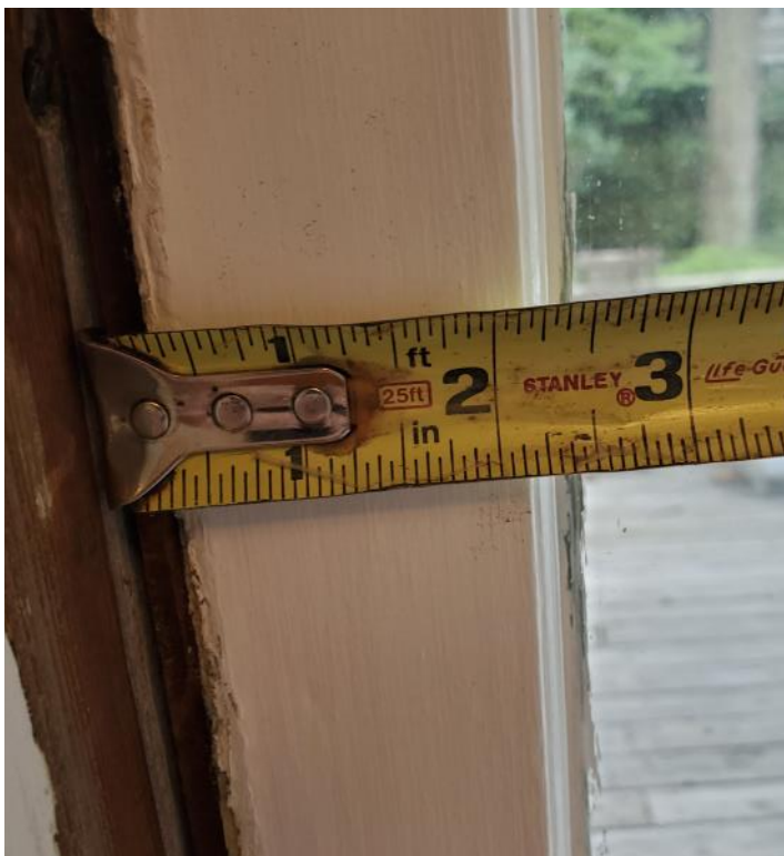
Left/right stiles: 2 3/8" + ~1/8" lateral travel space on each side
