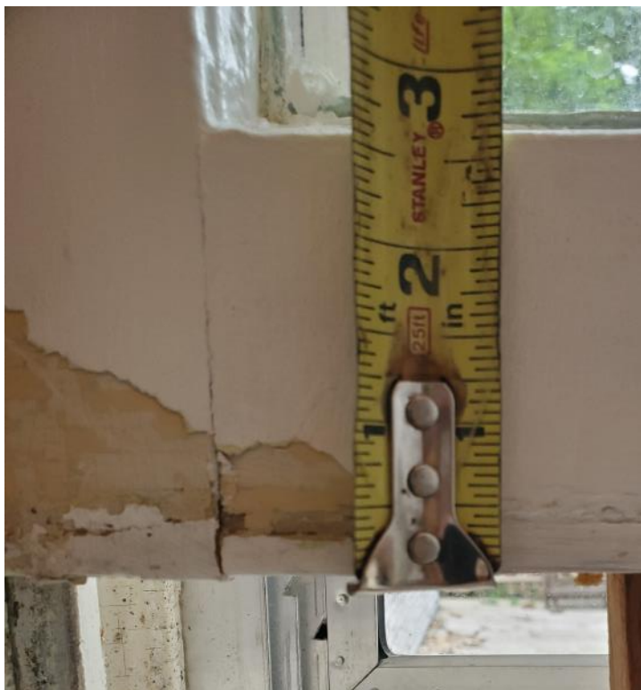
Bottom rail: 2 3/4" at interior edge of sloped sill
