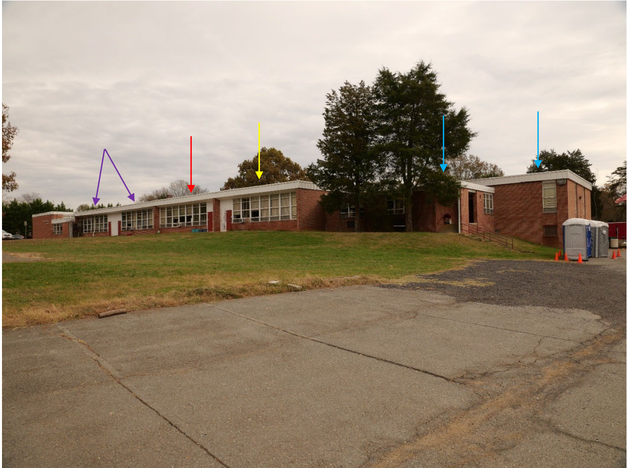
Figure 4: View of the north (façade) and west elevation looking southeast. The purple arrows point to the original classroom wing (1952), the red arrow points to the first classroom addition (1954), the yellow arrow points to the second classroom addition (1961), and the blue arrows point to the library and services wing (1969).
