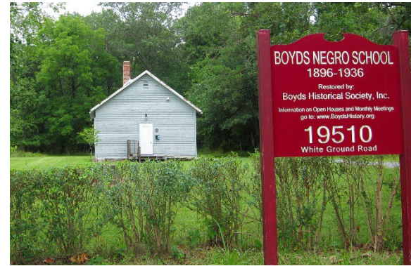
The Boyds Negro School located in the southern section of the Boyds Historic District
