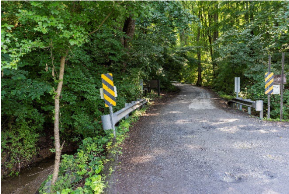
One-lane bridge leading to the C&O Canal parking lot
