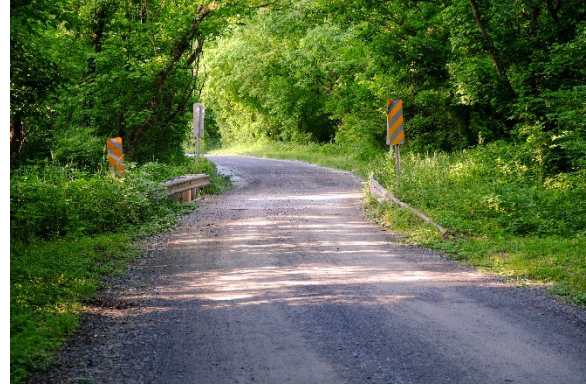
The northernmost one-lane bridge on Sycamore Landing Road
