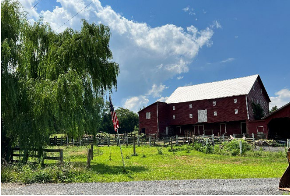
View from Sugarland Road just west of Dry Seneca Creek
