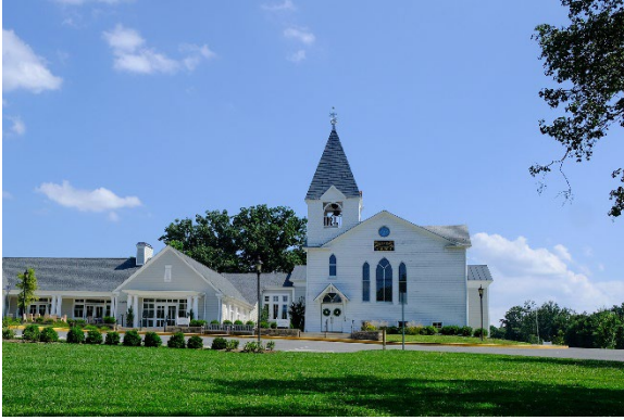
Darnestown Presbyterian Church located at the northern end of Turkey Foot Road
