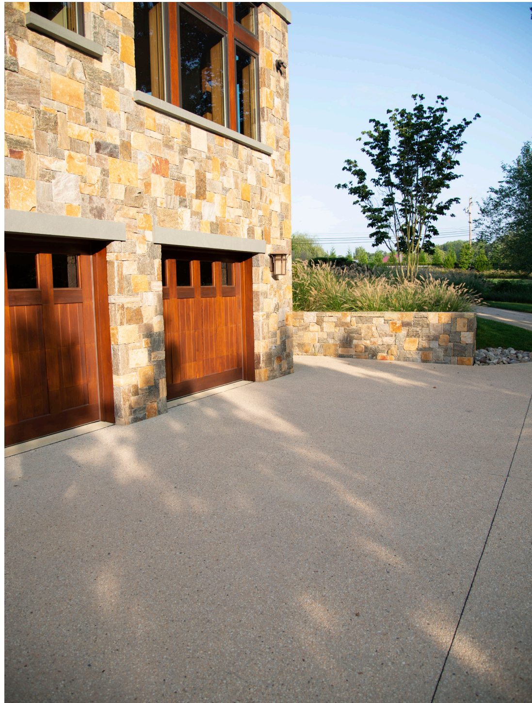
JANUARY 2021 SUBMISSION (APPROVED) - CONCRETE PAVING
