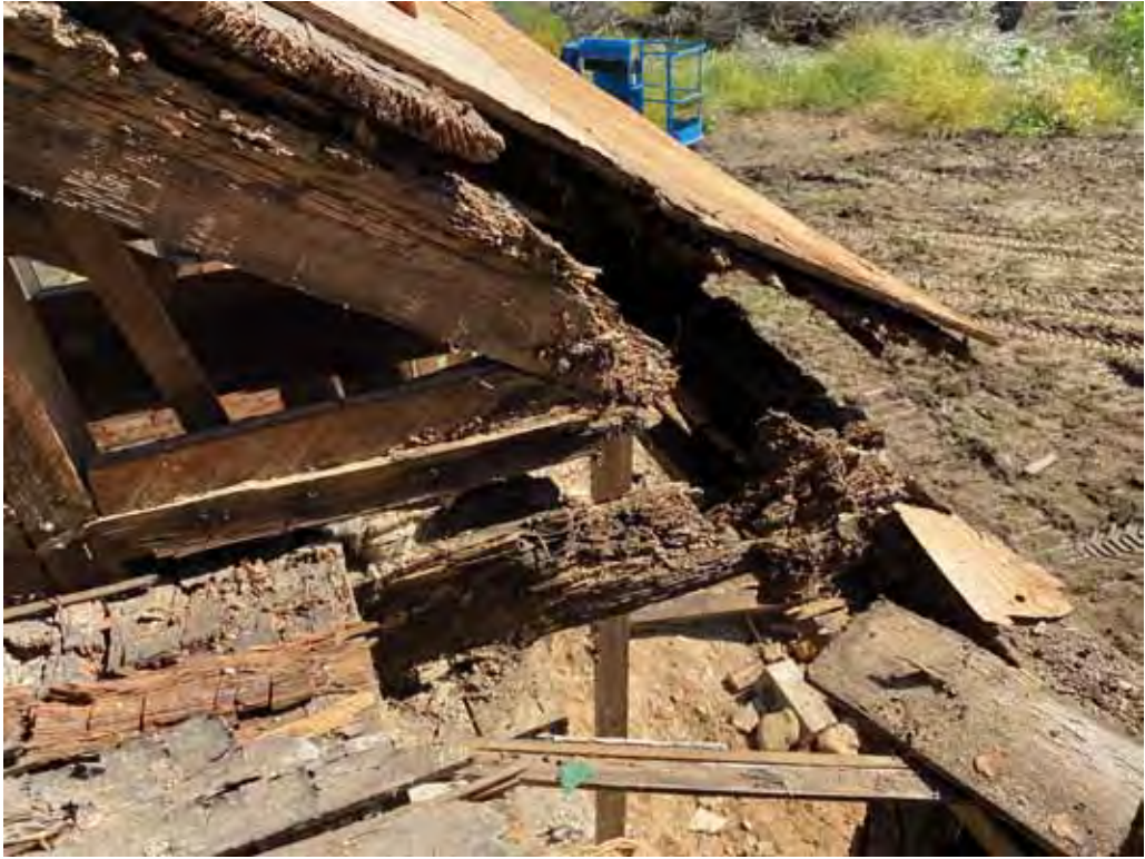
4 ROTTED STRUCTURE AT COLLAPSED SHED ROOF AT BATHRMS
