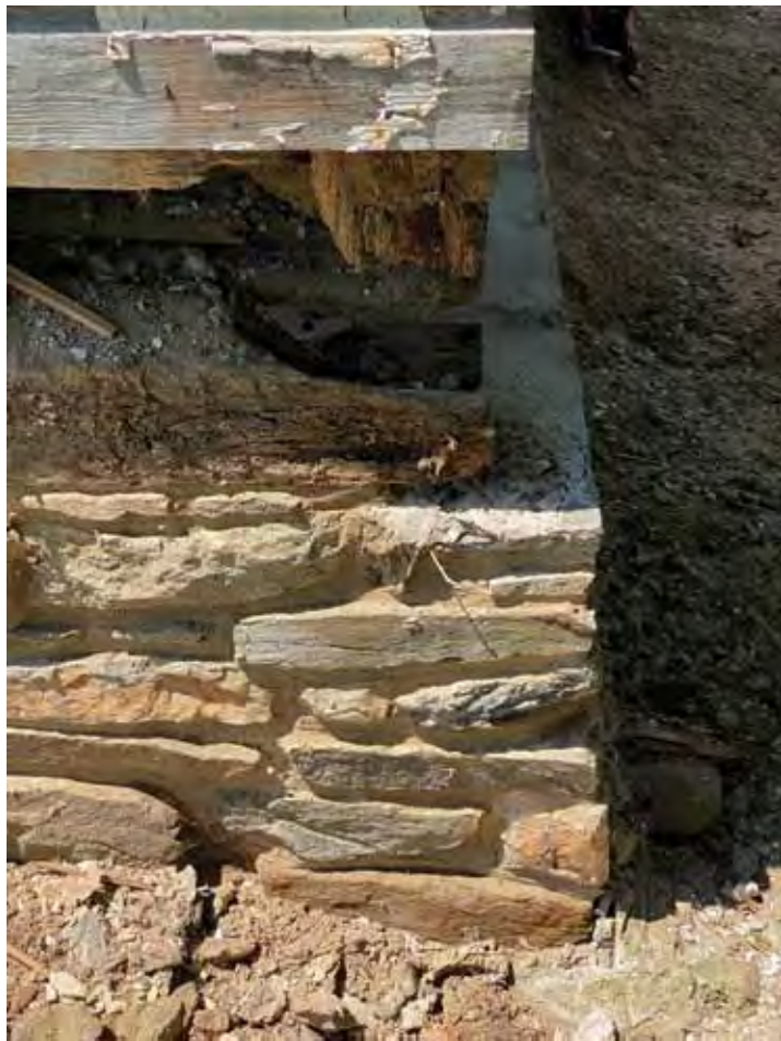
3 ROTTED SILL + RESTORED FNDTN AT NW
