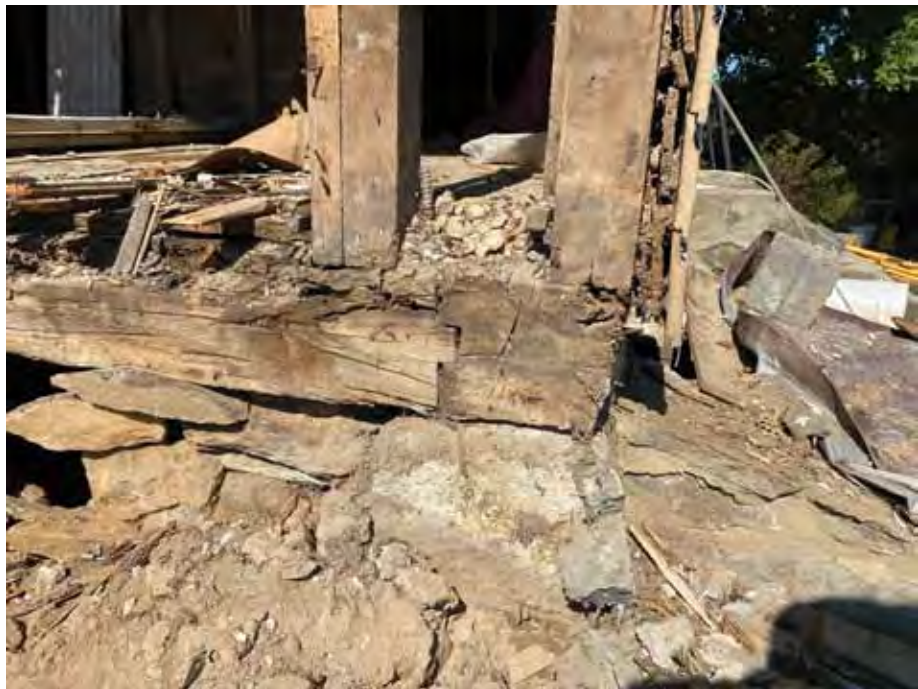
6 DEGRADED ORIGINAL FNDTN + STRUCTURE AT SE
