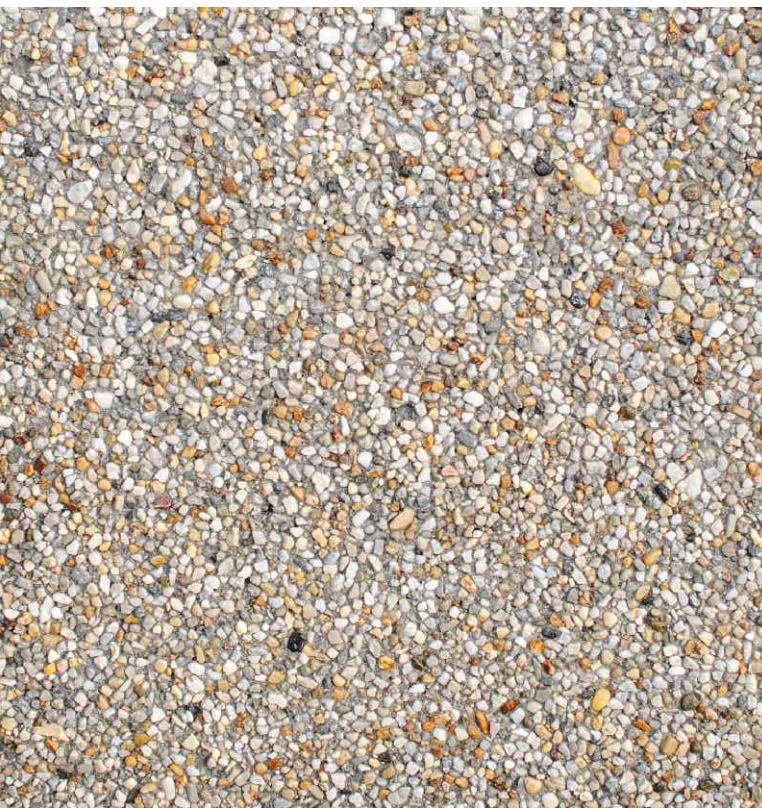
EXPOSED AGGREGATE CONCRETE TO BE REPLACED IN-KIND IN DRIVEWAY AND PARKING COURT
