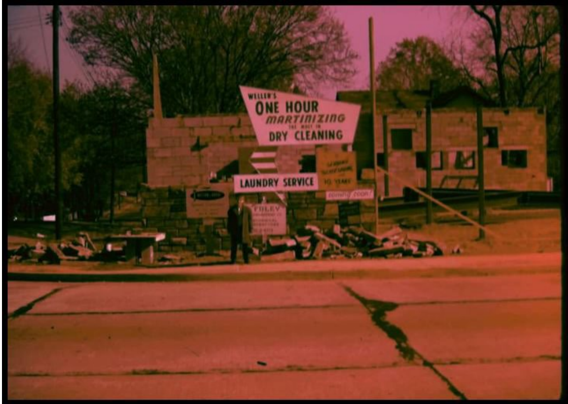
Figure 1: View of the Weller's Dry Cleaning under construction, ca. 1961. Note the sign that reads "Weller's One Hour Martinizing." The concrete block wall on the rear elevation and the stone veneer on the front elevation are visible.
