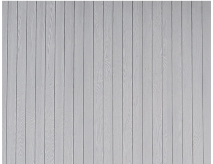
Figure 6: Typical tongue and groove siding.
