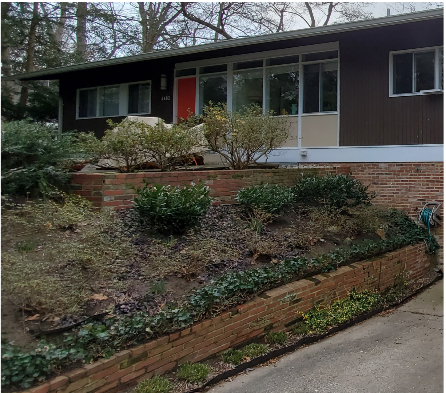
Figure 46: Example of brick retaining walls.
