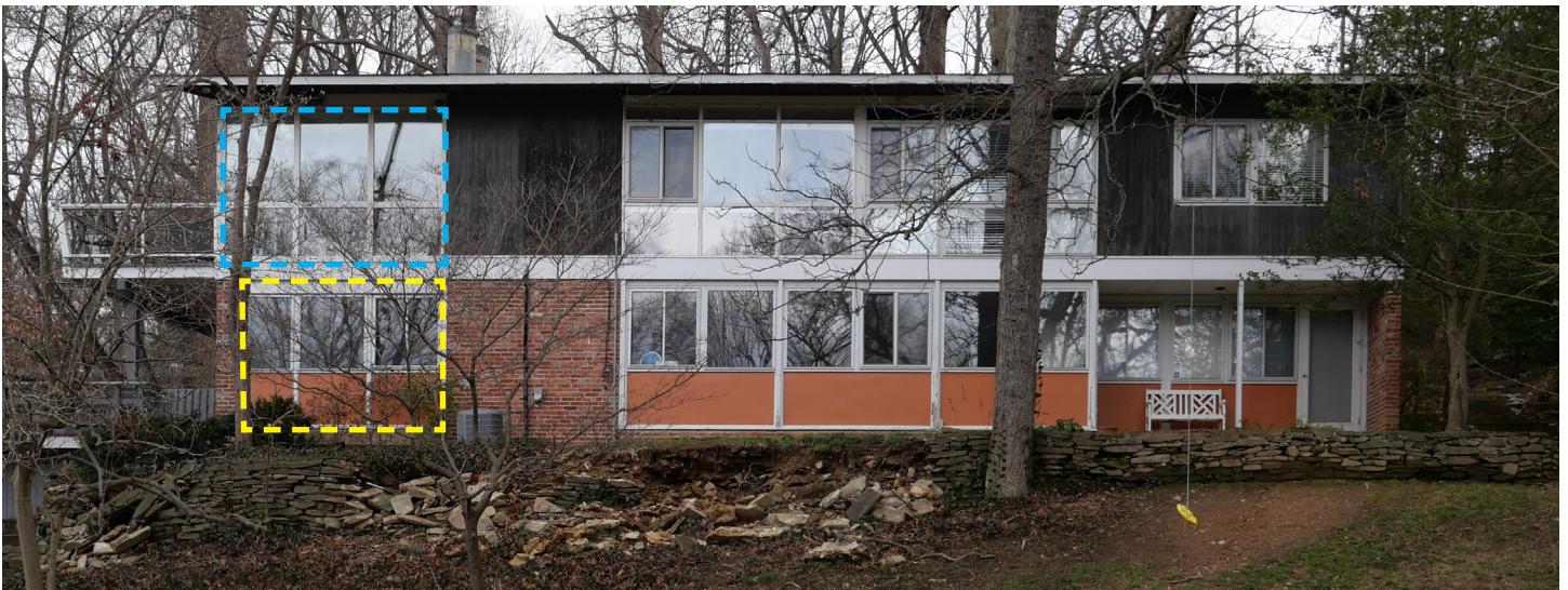
Figure 20: The dwelling at 6525 Wiscasset Road includes the infill of the open patio (dashed yellow line) on the first story and enclosure of a screened-in porch (dashed blue line) on the second story.
