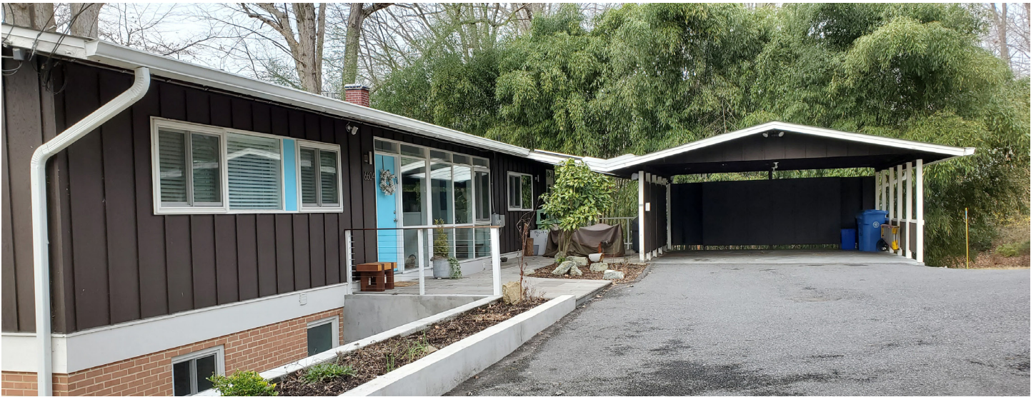
Figure 35: Example of an semi-attached carport with breezeway.
