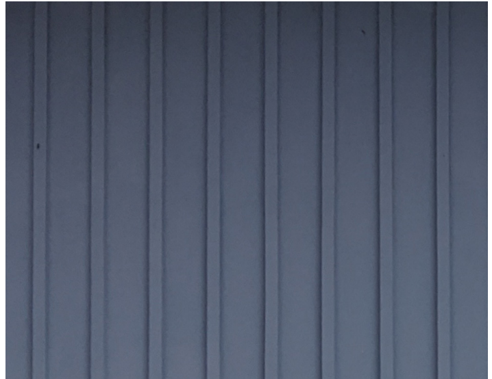
Figure 5: Typical board and batten siding.
