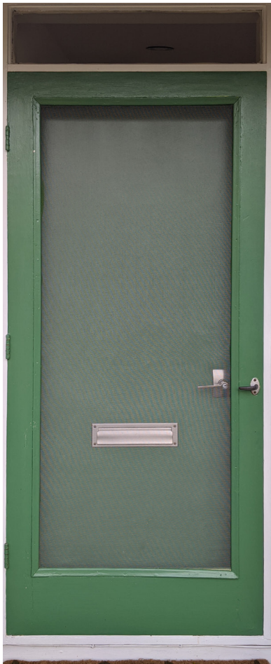
Figure 11: Example of an entrance door with screen door.
