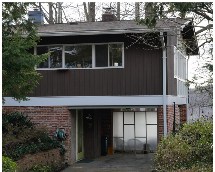
Figure 34: Example of an attached below-grade carport.
