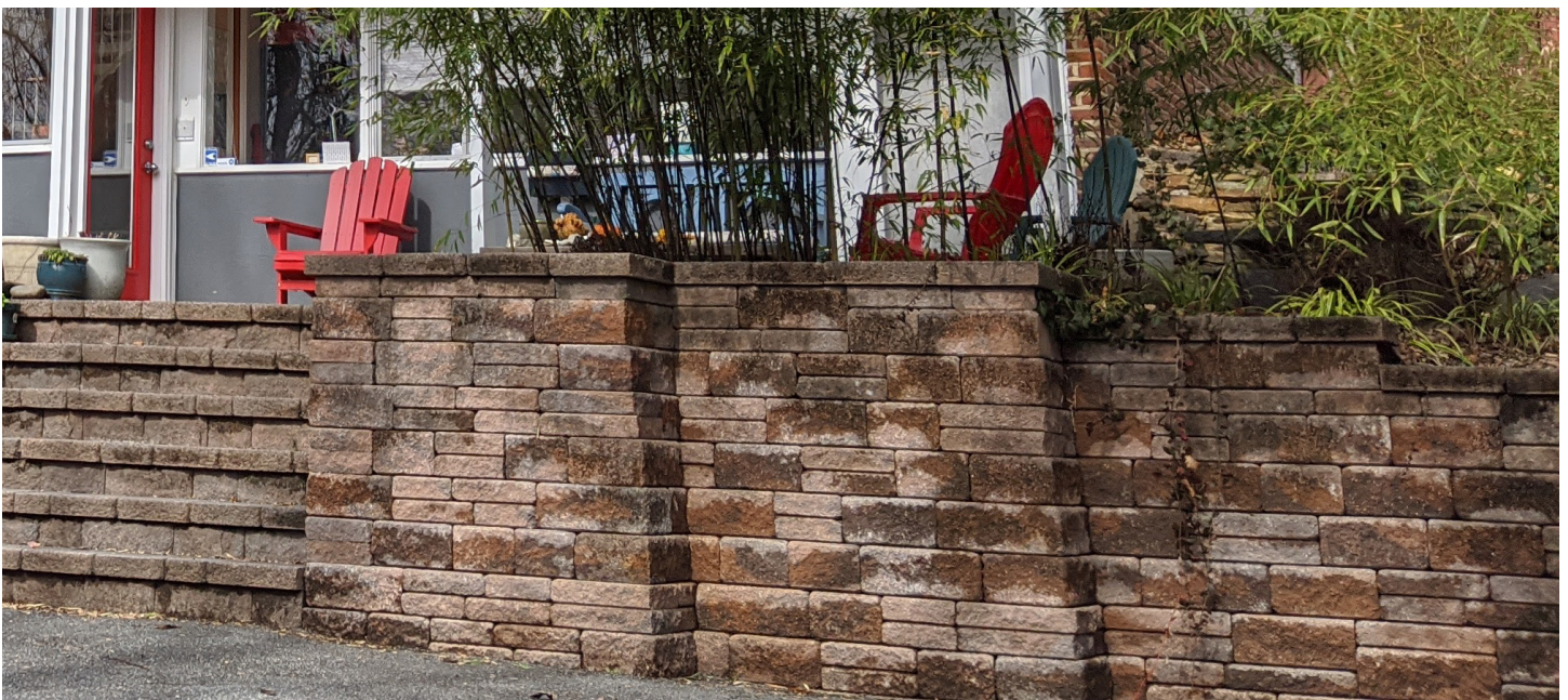
Figure 48: Example of masonry veneer walls.
