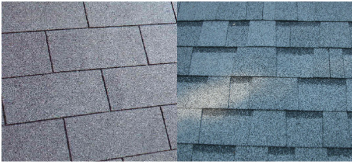
Figure 17: A comparison of three-tab asphalt shingles (left) and architectural asphalt shingle (right). Both styles of shingle can be utilized as an in-kind replacement without a HAWP.
