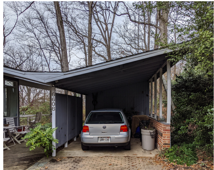
Figure 33: Example of a semi-attached carport with breezeway.
