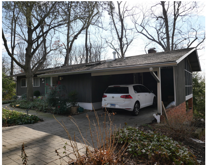
Figure 32: Example of an attached carport.
