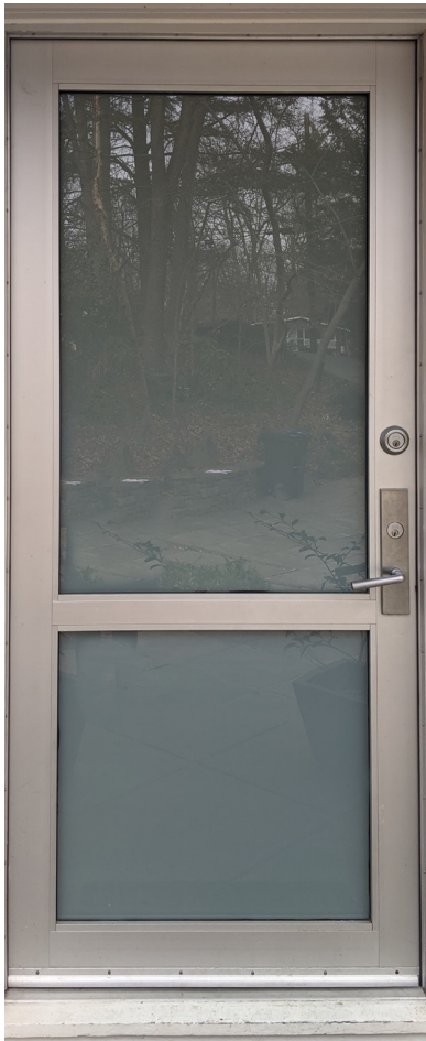
Figure 13: Example of a two-light, replacement entrance door.
