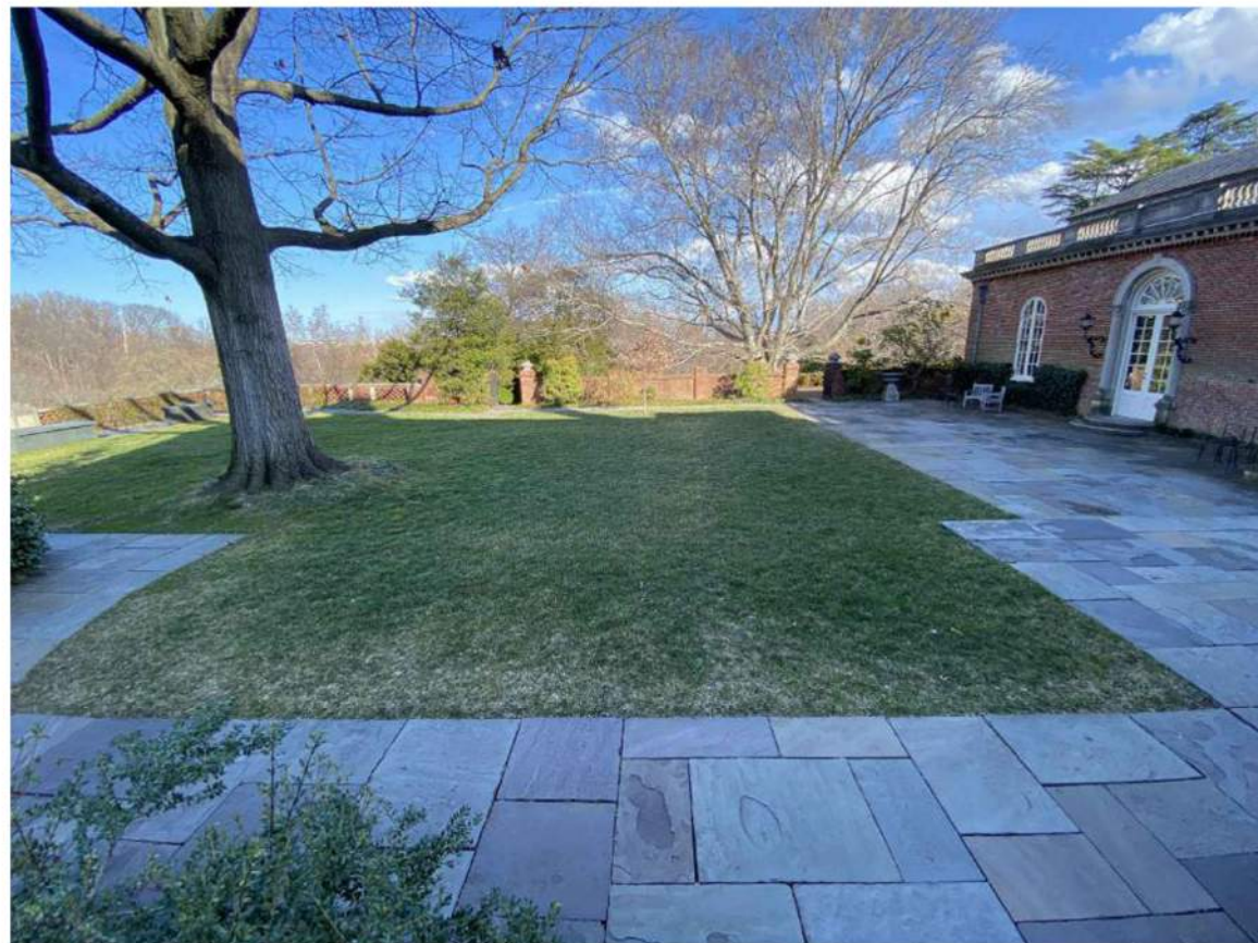
WORK ITEM #7 ACCESSIBLE EAST PATIO & WORK ITEM #8 ACCESSIBLE NORTH PLAZA: UNEVEN AND DAMAGED PAVERS PROPOSED EAST PATIO AND EXISTING NORTH PATIO RENEWAL WITH MORTAR SET BLUESTONE PAVERS
