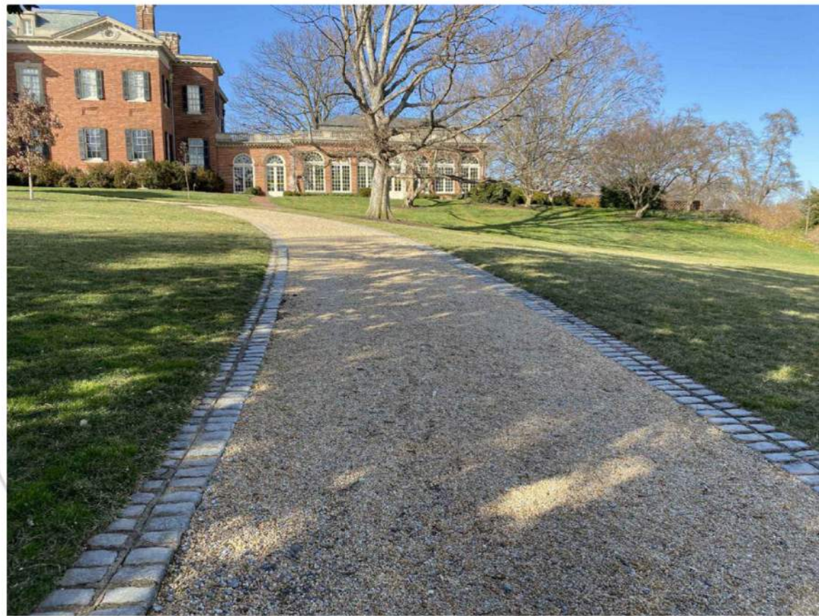
WORK ITEM #1 DRIVE ALONG SOUTH FAÇADE & WORK ITEM #2 DRIVE TURNAROUND PROPOSED SEEDED AGGREGATE CONCRETE DRIVEWAY WITH MORTAR SET COBBLE EDGE
