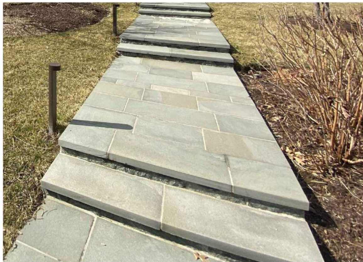
WORK ITEM #9 SUNROOM WEST PATIO AND STEPS TO GRADE PROPOSED STEPS AND NEW WEST PATIO WITH MORTAR SET BLUESTONE PAVERS
