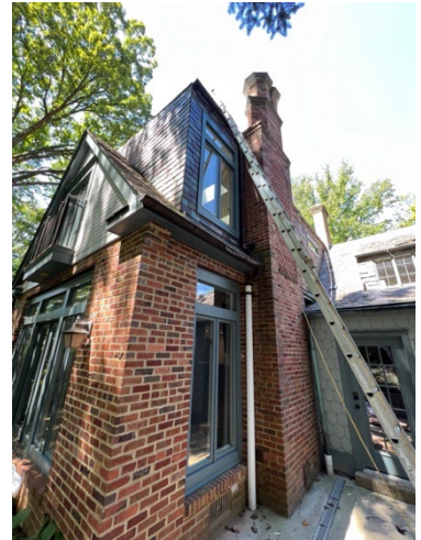
Figure 10 - Out of Code Downspout next to utility area
