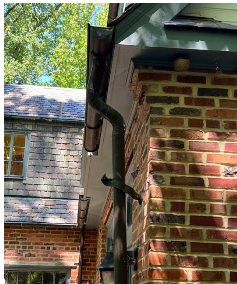
Figure 15 - downspout damage
