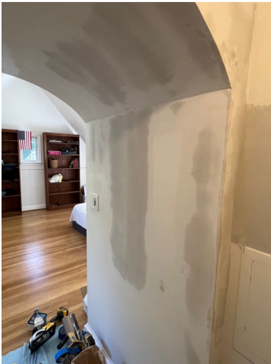
Figure 4: Water damage from roof and gutters - 2nd story
