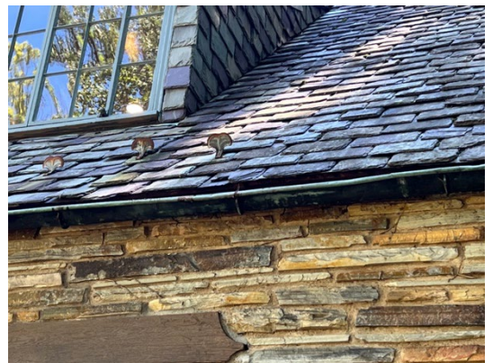
Figure 6 - Bent Gutter leading to water ingress
