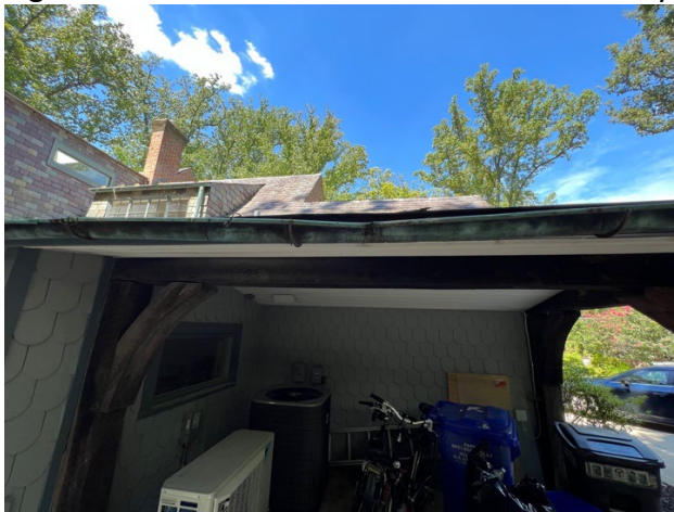
Figure 12 - Bent Gutter at Utility Area
