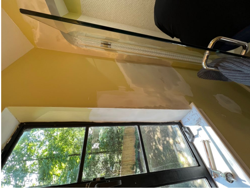
Figure 3: Bathroom water damage from roof & gutters
