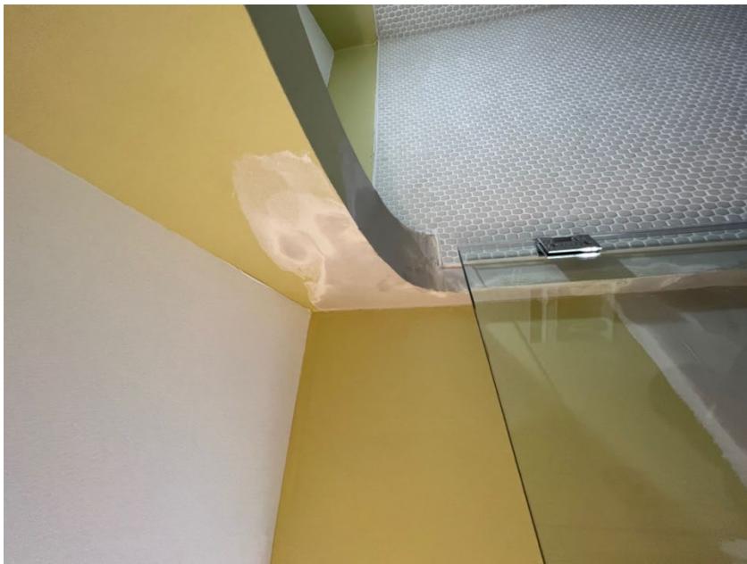
Figure 2 - 2nd Story Bathroom Water Damage from Gutters/Roof
