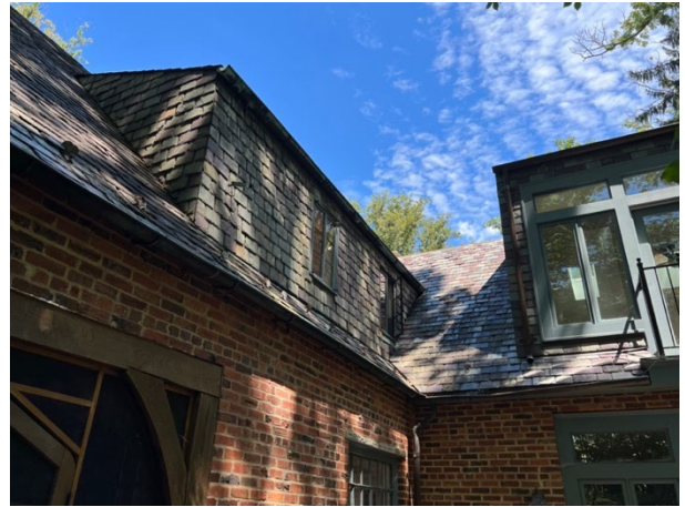
Figure 13 - bent gutters
