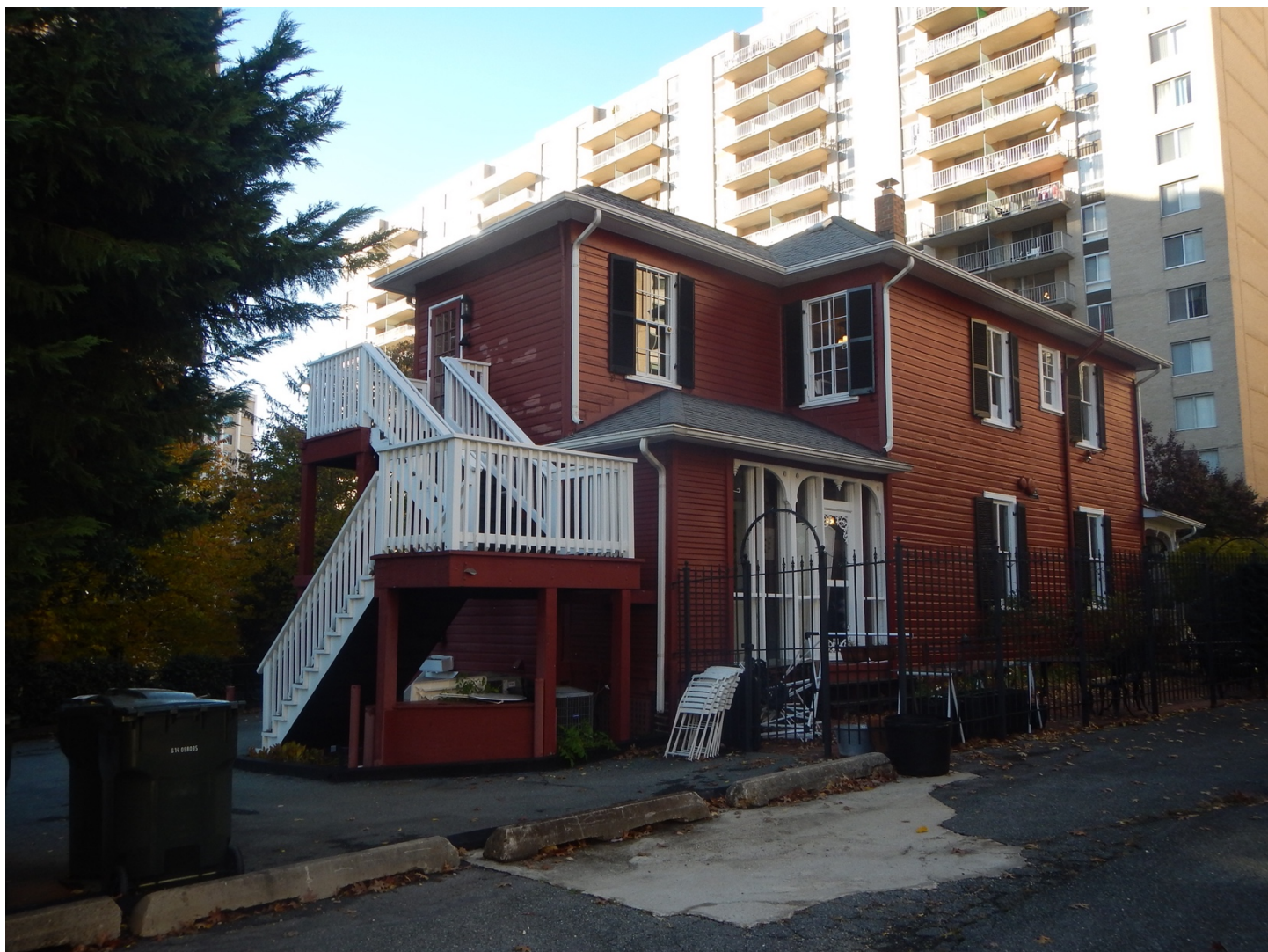
Figure 8. View of Rear of Joseph F. Pyles House, Facing Northwest (November 15, 2021).
