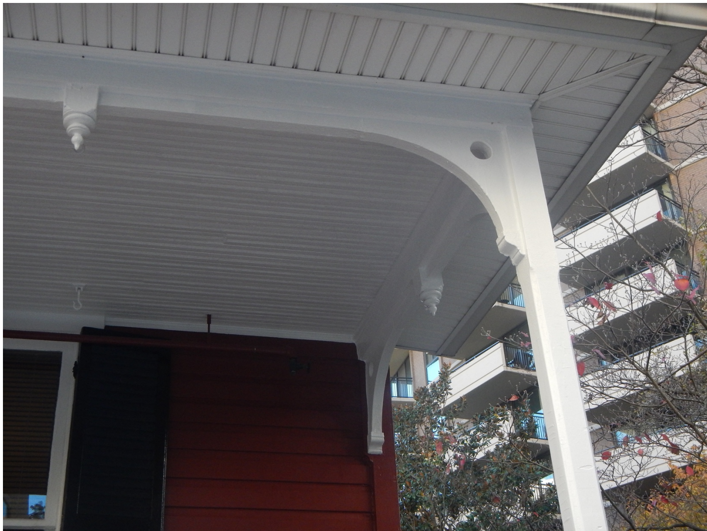
Figure 15. Detail of Trim and Pendant Decoration on Front Porch of Joseph F. Pyles House, Facing South (November 15, 2021).
