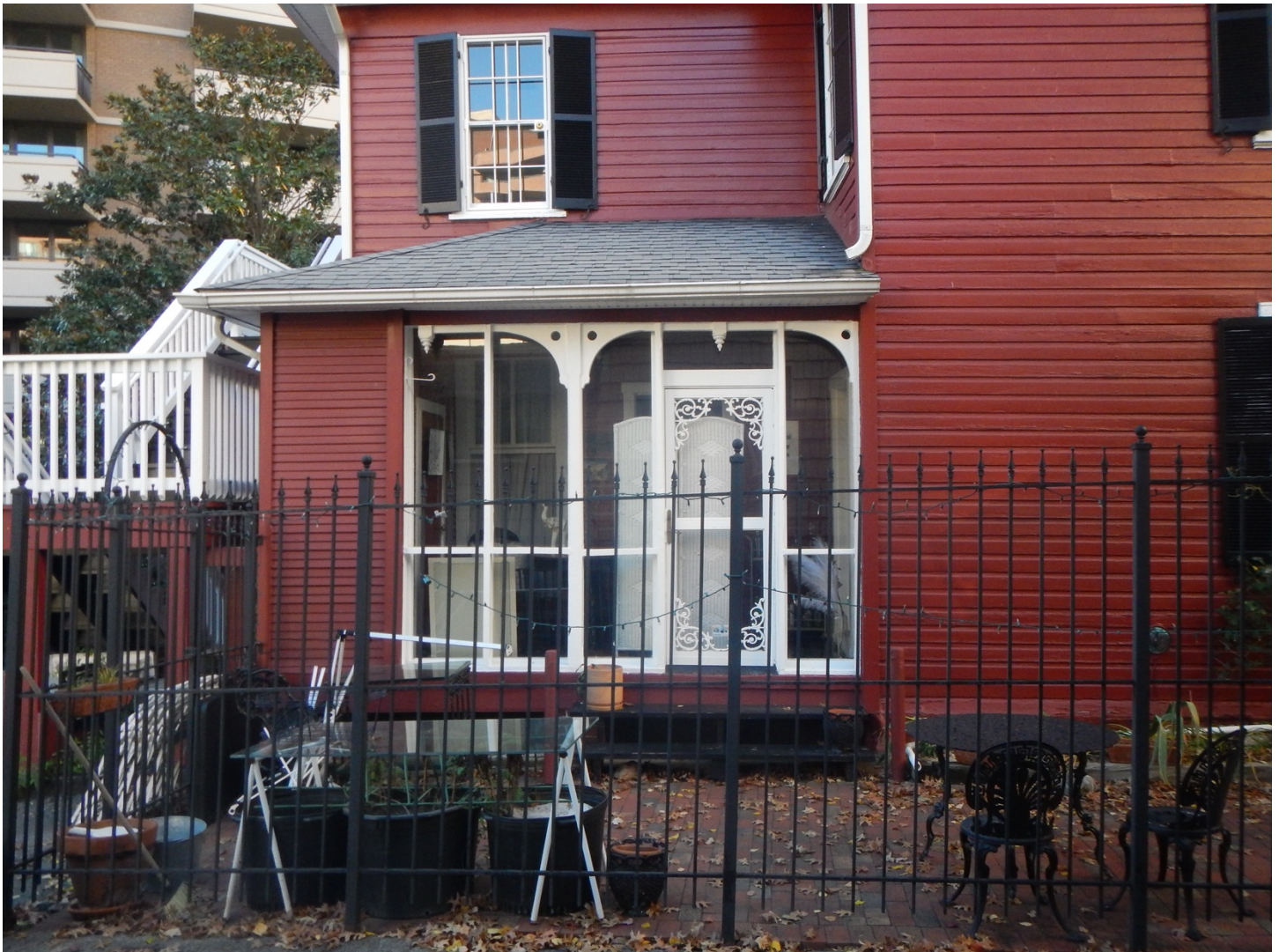
Figure 9. Detail of Enclosed Porch at Rear of Joseph F. Pyles House, Facing South (November 15, 2021).
