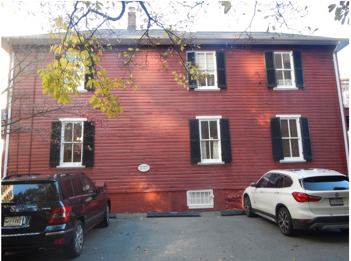
Figure 12. West Façade of Joseph F. Pyles House Showing Concrete Block and Stone Foundation Materials, Facing East (November 15, 2021).
