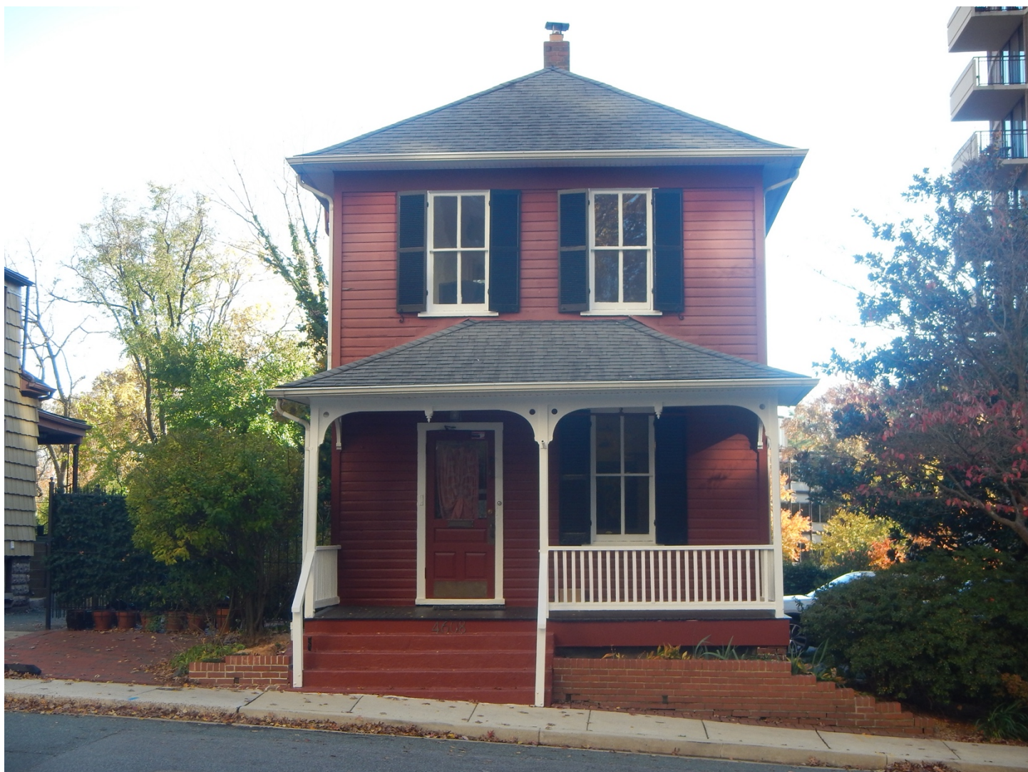
Figure 5. North Façade of Joseph F. Pyles House, Facing South (November 15, 2021).
