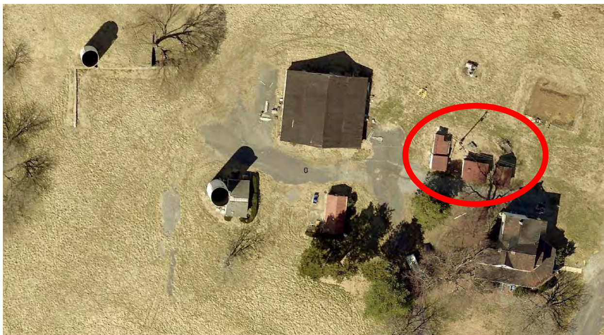
Figure 2: Detail showing the house and farm structures. Outbuildings proposed for demolition circled.
