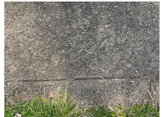
existing exposed aggregate finish
