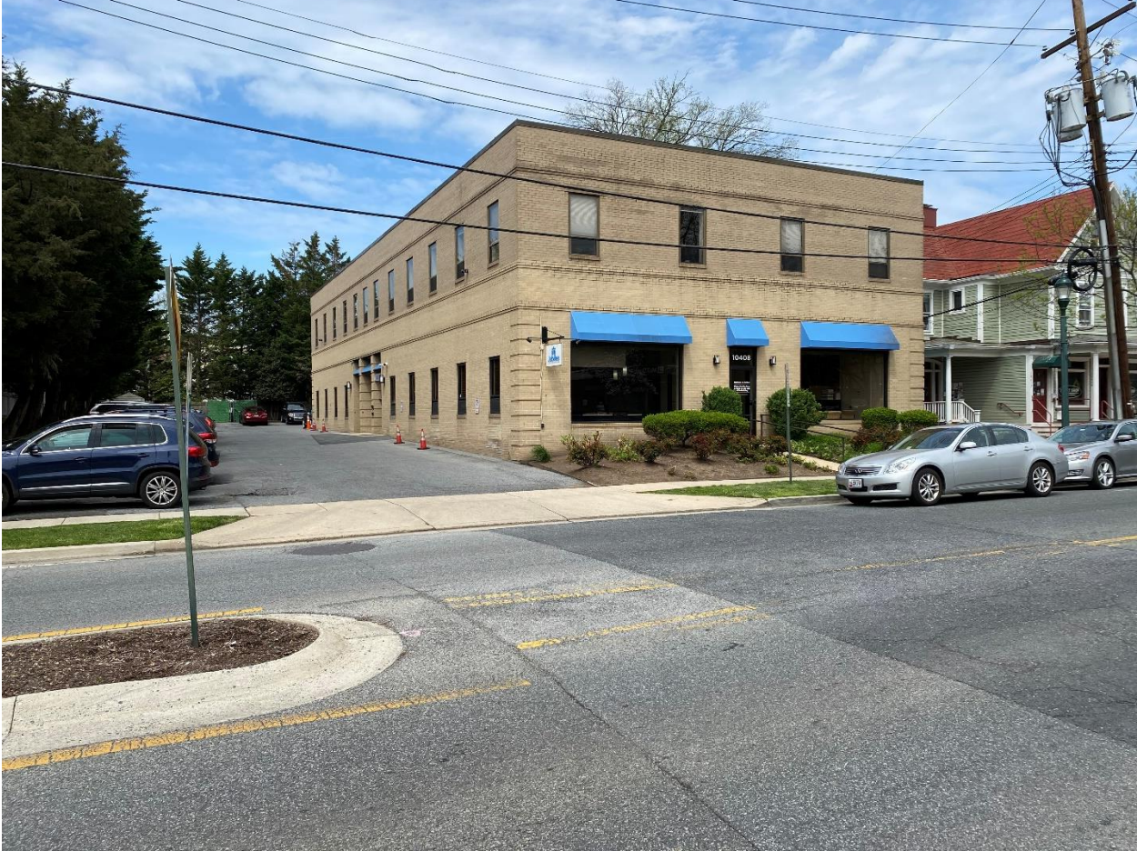
Figure 2: Looking along the south and east elevations of the subject property.
