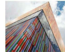
Patterns on this glass building reduce the likelihood of bird collisions. Source: naturalimages.net
