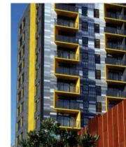
Balconies provide shadows and limit reflections on glass to deter birds. Source: Merchant Quarter Condominiums
