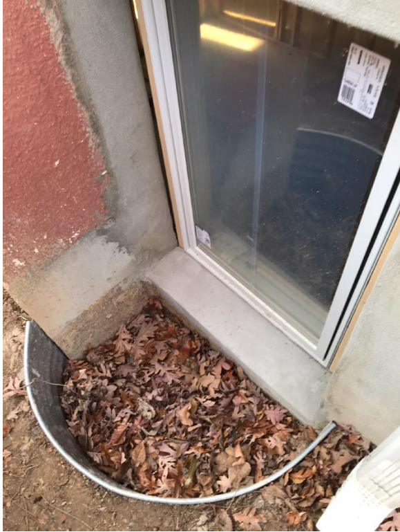
Fig. 6: Staff's December 2021 site visit photograph, showing the unpermitted basement level egress window with window well on the east/left side of the historic house.
