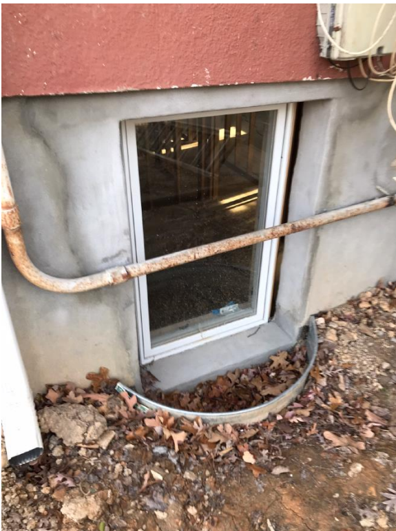
Fig. 5: Staff's December 2021 site visit photograph, showing the unpermitted basement level egress window with window well on the west/right side of the historic house.
