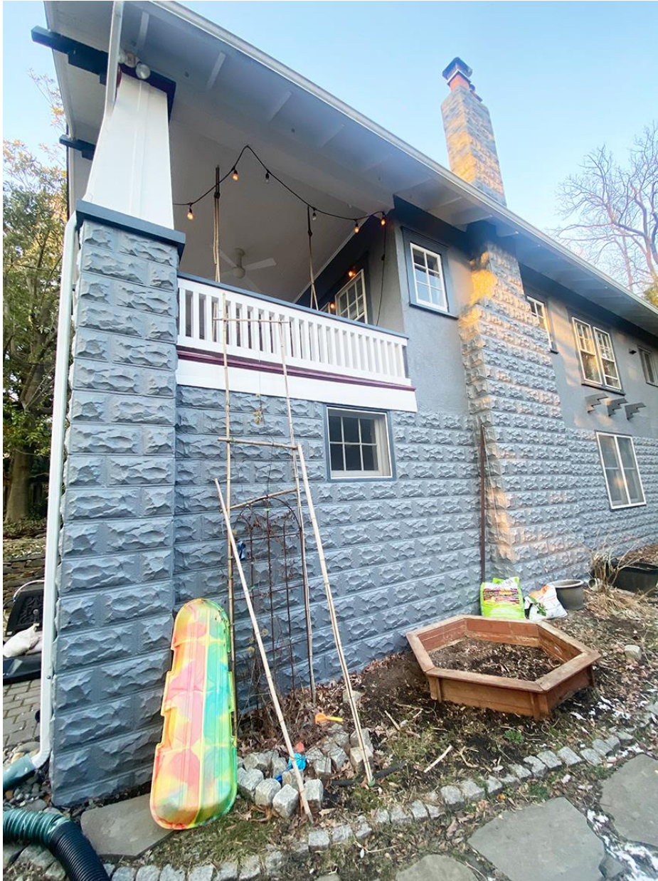
Fig. 3: South/right side of the historic house and original attached garage, showing the character-defining rusticated concrete block.
