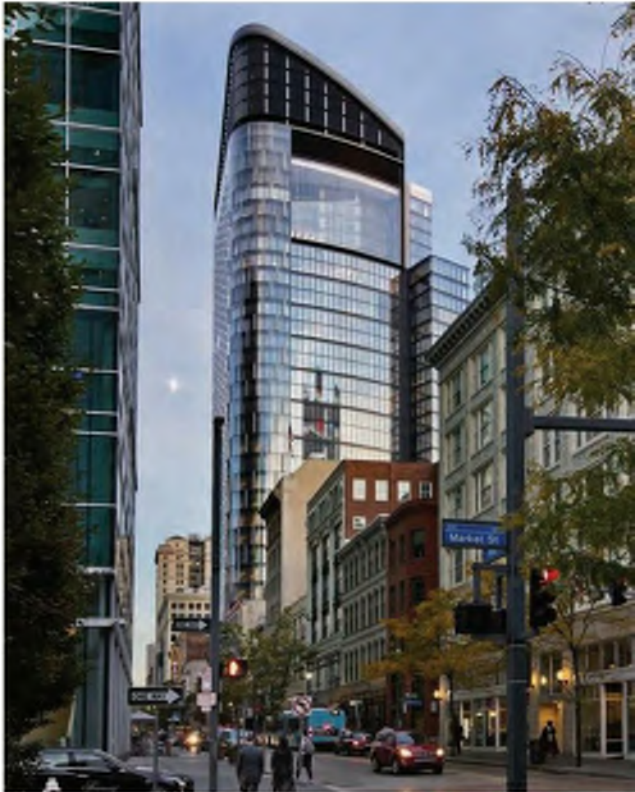
The form of the tower top for this Pittsburgh office building is part of the energy efficient solar chimney design. Source: Gensler
