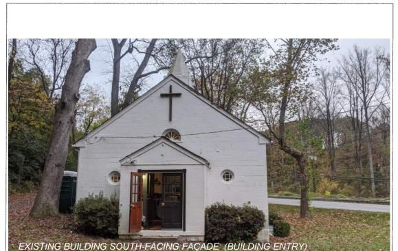
BUILDING/FAÇADE TO BE LIFTED FOR FLOOD MITIGATION AND Detail: RECLAD TO MATCH ORIGINAL(REAR) STRUCTURE
