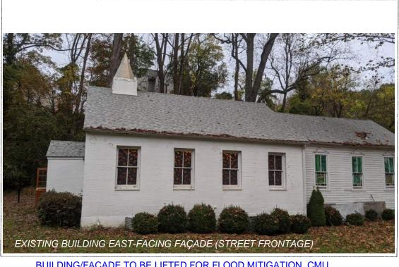
BUILDING/FAÇADE TO BE LIFTED FOR FLOOD MITIGATION, CMU Detail:\_(FRONT) TO BE RECLAD TO MATCH ORIGINAL(REAR) STRUCTURE, AND\_\_\_\_\_ WATER-DAMAGED FOUNDATION AREA TO BE REPAIRED/REPLACED
