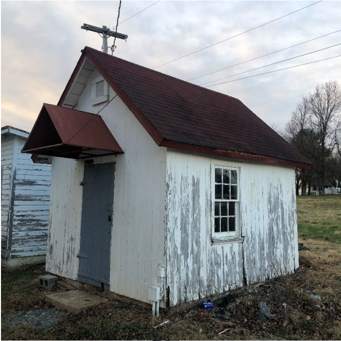
Current photographs of Pump House, Handyman Room and Hen House:
