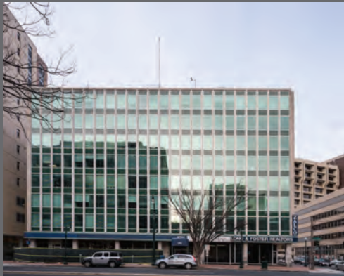
American National Bank Building, 2012. Source: Montgomery Planning Archives.
