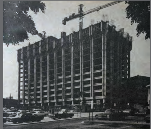
Montgomery Center, under construction. Source: Suburban Record.
