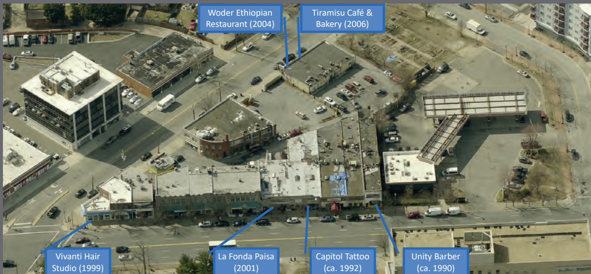
Aerial view of Georgia Avenue and Eastern Avenue. Source: Pictometry.
