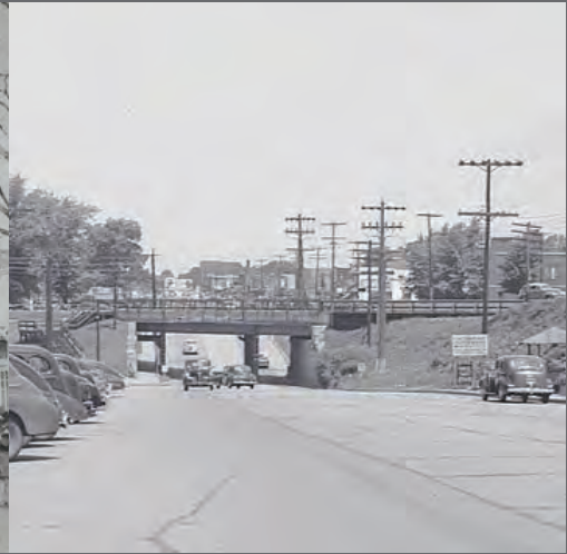
Georgia Avenue Viaduct, 1925.
