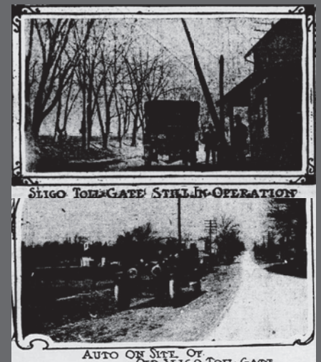
Toll house on Georgia Avenue still in operation in 1912 (top) and new macadamized road at demolished toll house in 1914 (bottom). Source: Evening Star.
