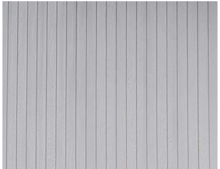
Figure 6: Typical tongue and groove siding.
