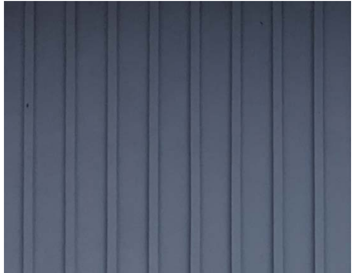
Figure 5: Typical board and batten siding.
