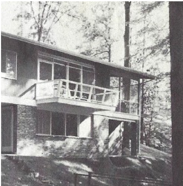
Figure 25: View of the rear elevation of the Highview model. Note the cantilevered balcony on the second-story of the building. The balcony extended the length of the window and door opening and consisted of a wood railing mounted to the flooring.
