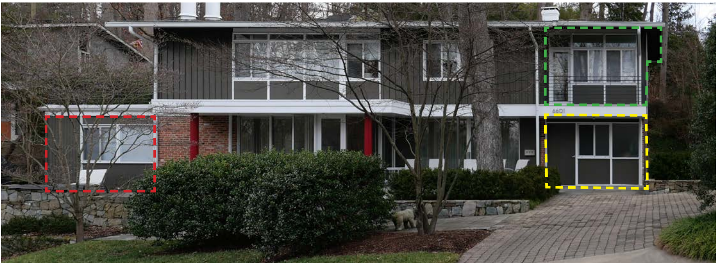
Figure 21: The dwelling at 6601 Virginia View Court includes the infill of the: 1) open patio (red dashed line), 2) carport (yellow dashed line); and 3) second-story addition and balcony above the carport (green dashed line).
