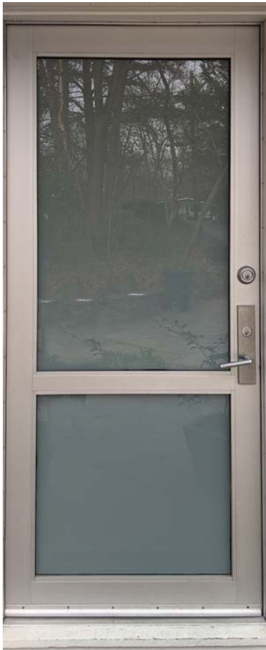
Figure 13: Example of a two-light, replacement entrance door.
