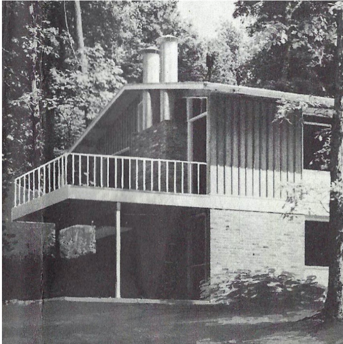
Figure 26: View of the front elevation of the Valleyview model. Note the partially cantilevered deck on the gable-end of the building. The deck railing may have been constructed of thin metal spindles, but all railing posts are deck-mounted allowing for an uninterrupted extension of the fascia board.
