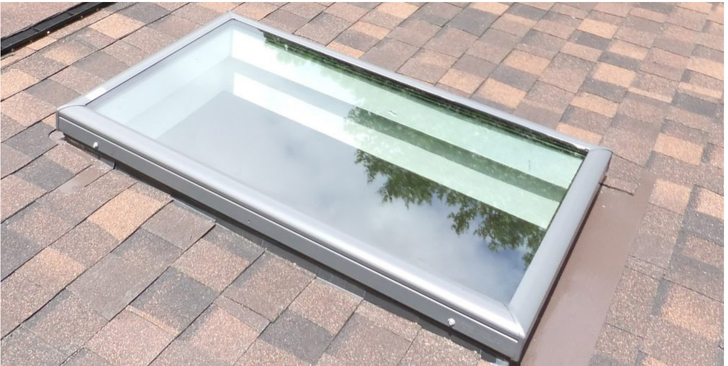
Figure 18: An example of a flat or low-profile skylight appropriate for installation.
