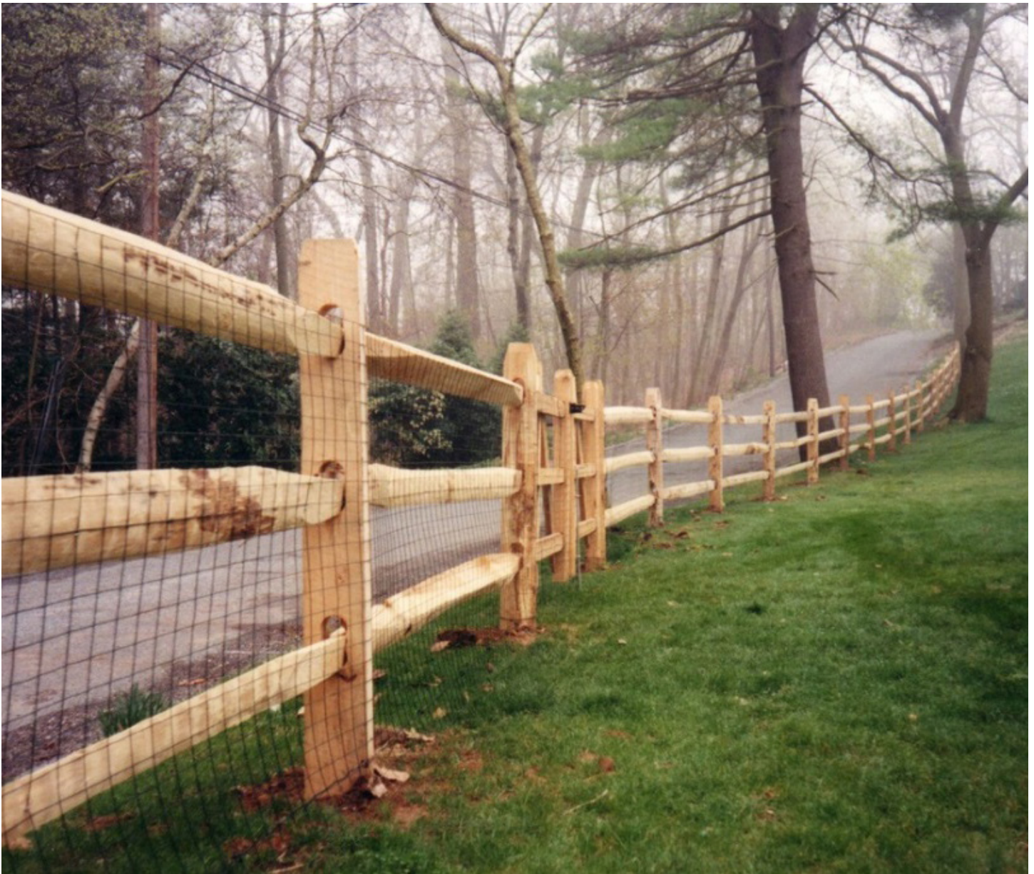
Figure 45: Example of a post and rail fence. The addition of wire/mesh is appropriate to increase containment capability.
