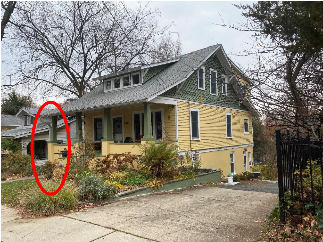
Figure 2: Note the severe lean in the left porch column.
