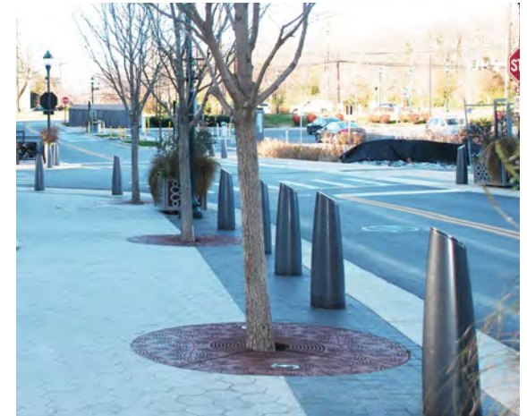
Figure 24: Tree Grate in Hardscape (Prose Street)
