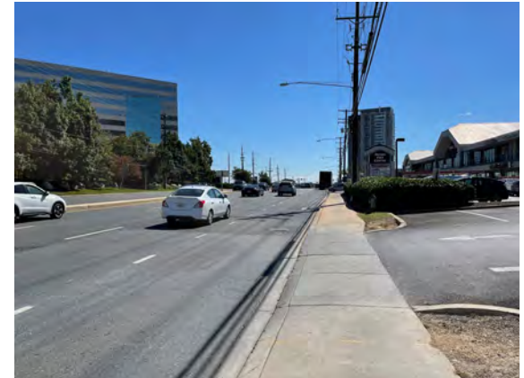
Figure 33: Example of an Undesirable PLOC score on Rockville Pike, with narrow sidewalks, no buffer from travel lanes and heavy traffic volumes.
