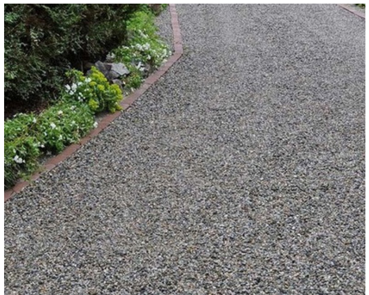
Figure 40: Example of a 3/8" crushed stone driveway.
