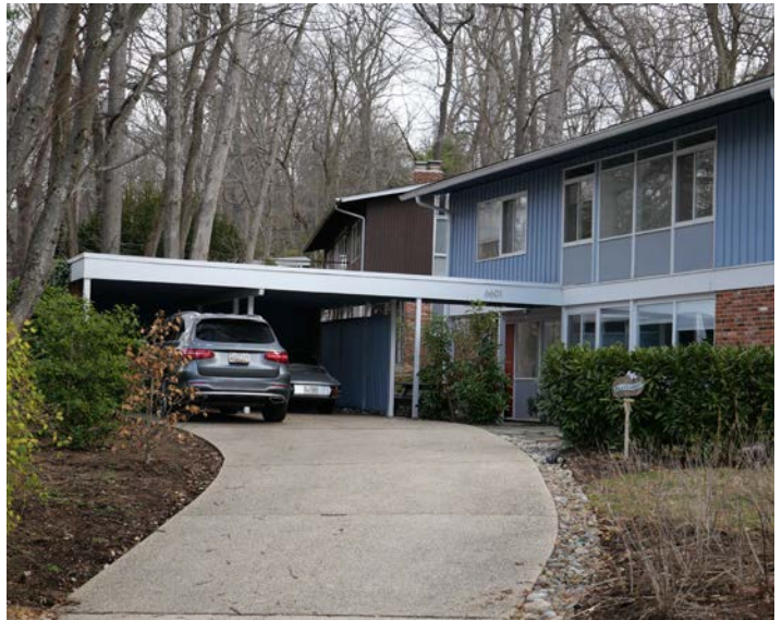
Figure 38: Example of a concrete driveway.
