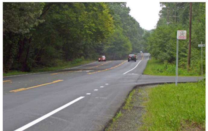
Road after four to three lane conversion
