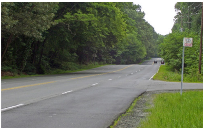
Road before four to three lane conversion
