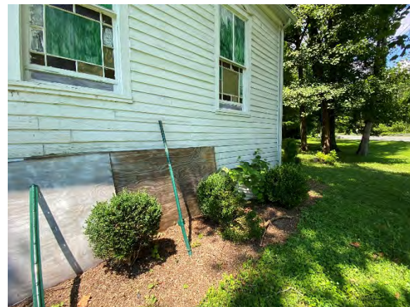
Figure 17: Detail of damaged foundation/partially exposed basement level at the original chapel volume.
