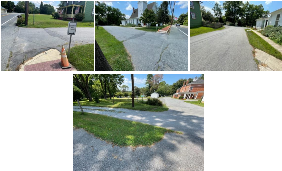
Figure A-2: Church Street Conditions (Note: Tar and Chip Surface will end where Gravel Begins)
