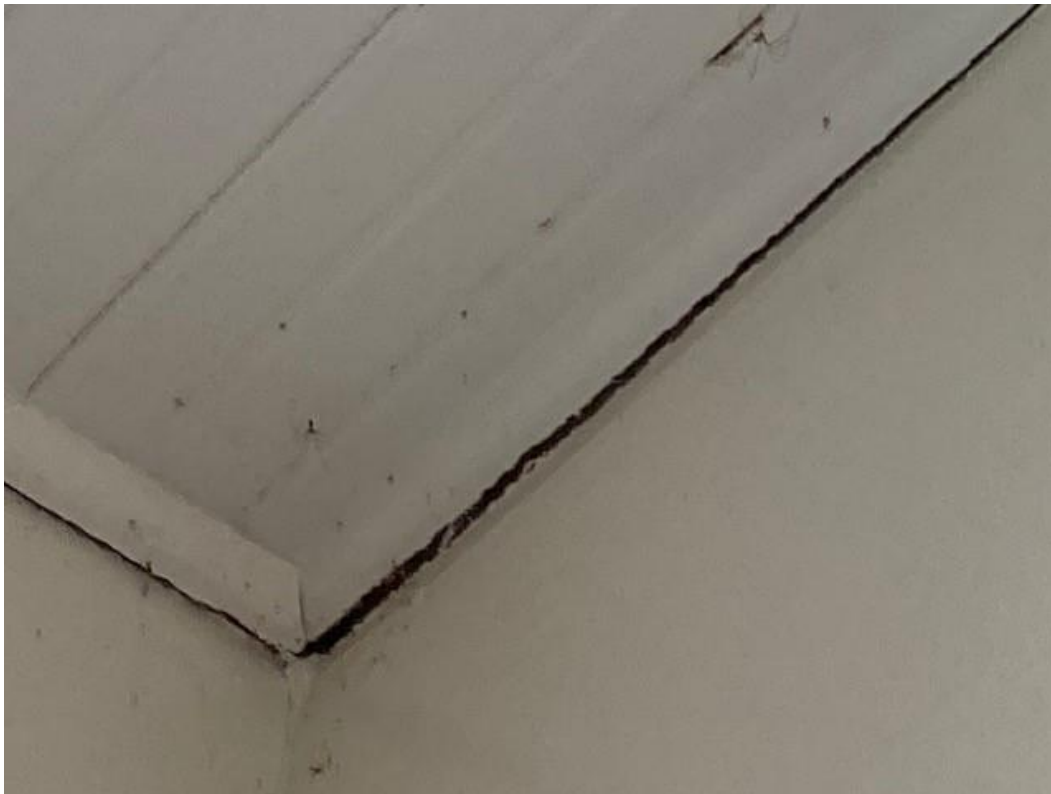
Walls separating from ceiling. These are not just cracks in the paint.
