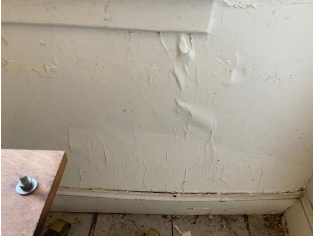
Bowing and separation of north wall under picture window.
