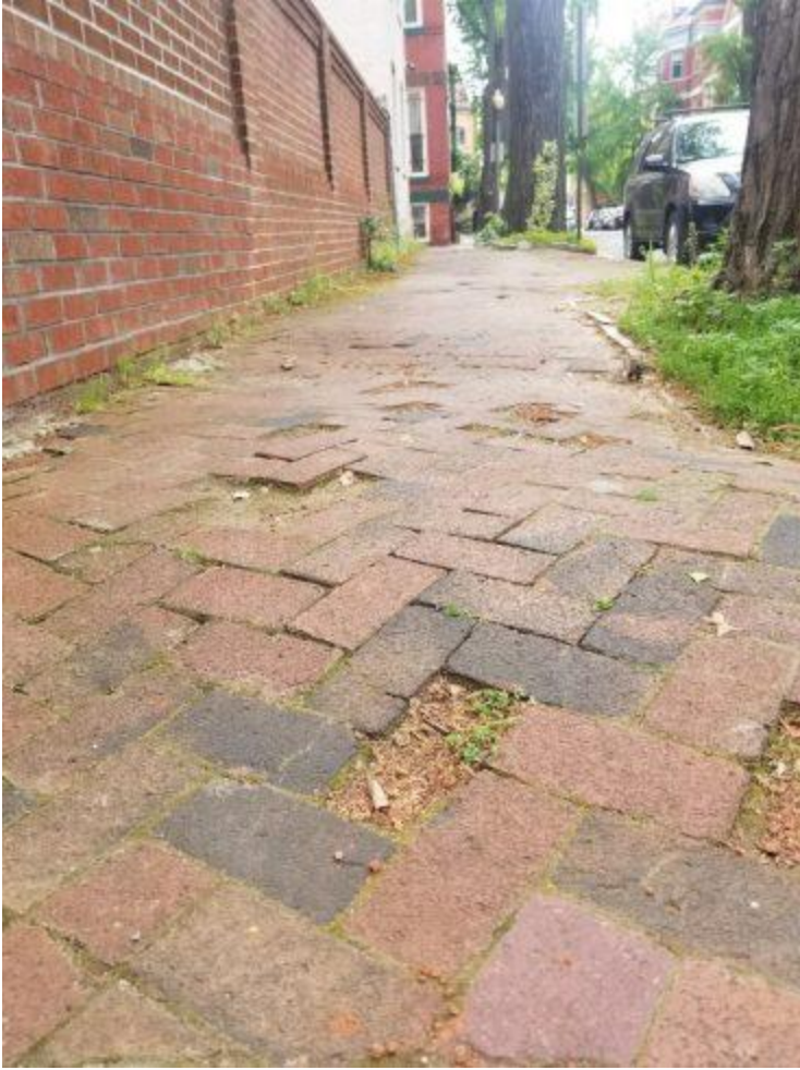
Brick sidewalks can also be tripping hazards if they are not well-maintained.
