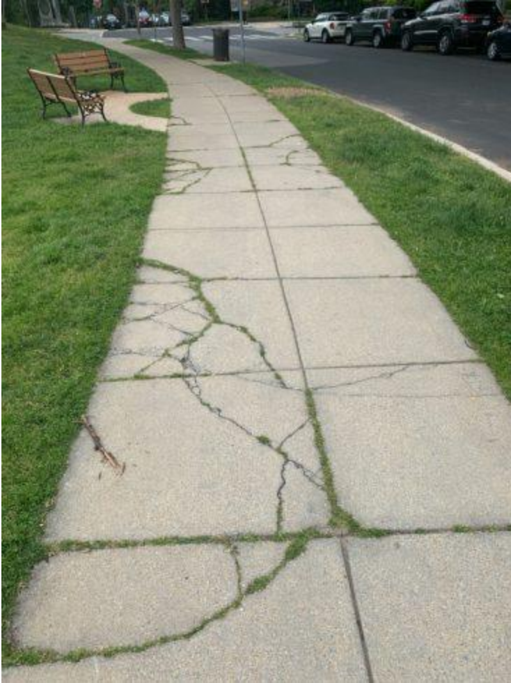
Sidewalk cracks can make a sidewalk inaccessible to people using wheelchairs. They are also a tripping hazard.
