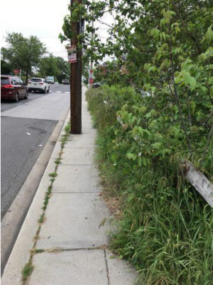
The telephone pole and overgrown vegetation make the sidewalk very narrow.
