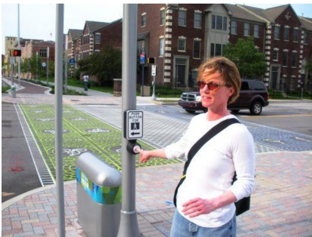
Pedestrians use the pushbutton to indicate they are waiting to cross. The pushbutton should be easy to reach.
