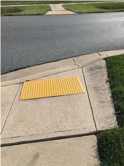
Detectable warning surfaces are textured bumps on curb ramps. They warn people that they are entering the roadway.
