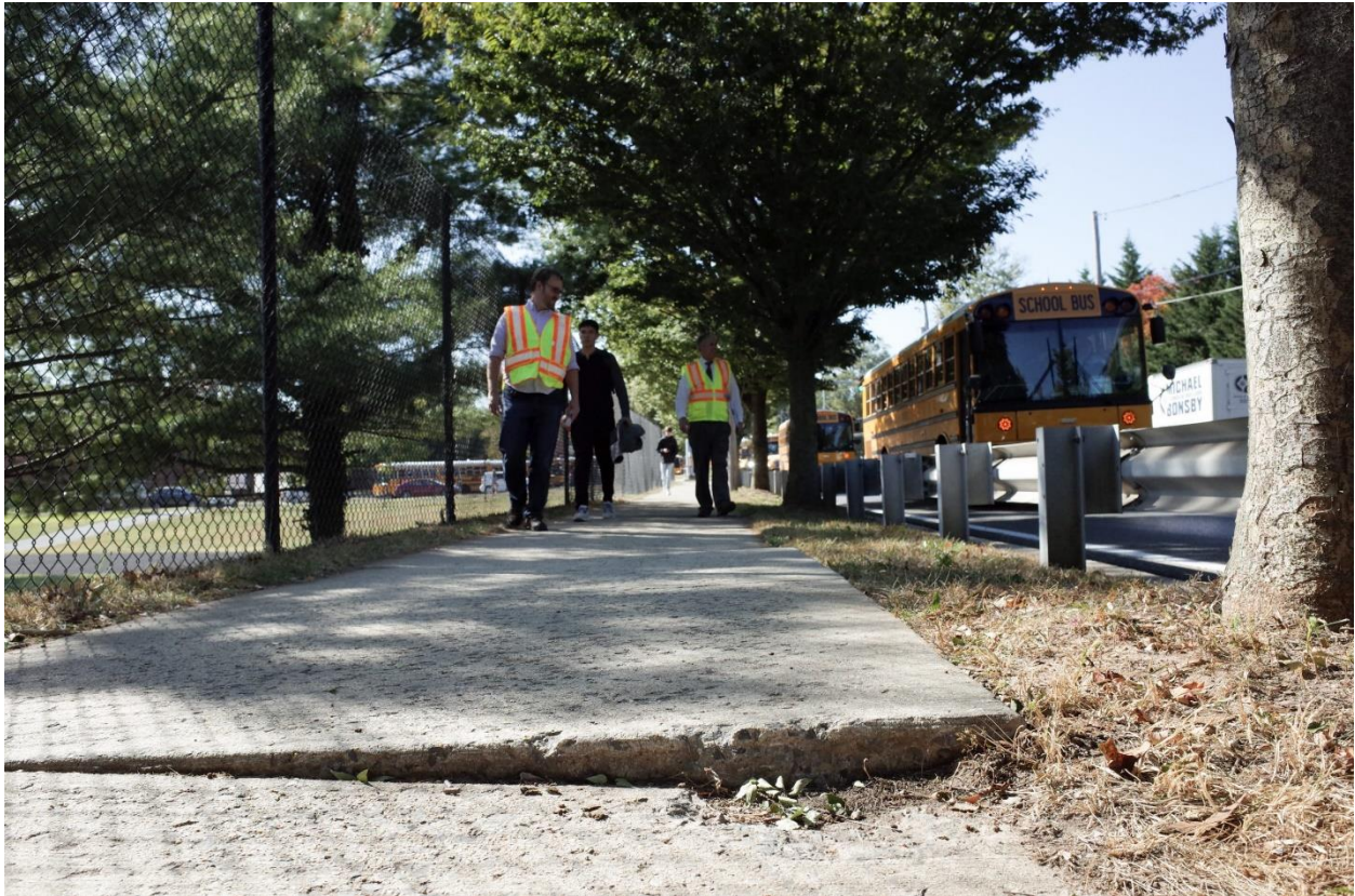
A sidewalk tripping hazard near a school in Ashton
