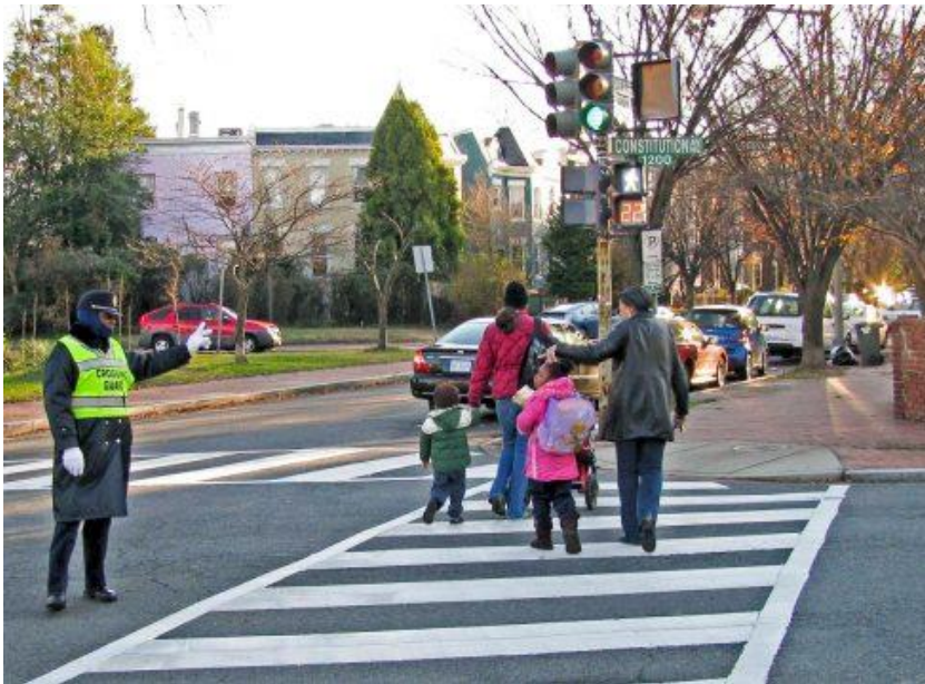
Continental and ladder-style crosswalks are considered high visibility crosswalks. They are easier for drivers to see and also more visible to pedestrians with low vision. Continental crosswalks are preferred by Montgomery County.
