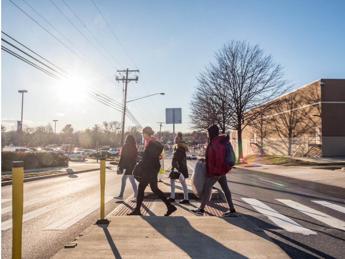
Pedestrians use a midblock crossing island in Aspen Hill
