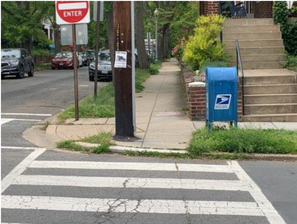
The lack of a curb ramp makes crossing difficult for people using wheelchairs, walkers, and strollers.
