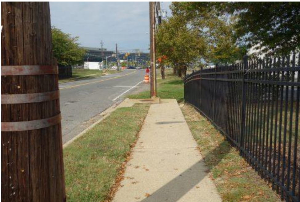
Disconnected sidewalks prevent access to destinations. Sidewalk gaps force pedestrians to cross the street or travel in the roadway.
