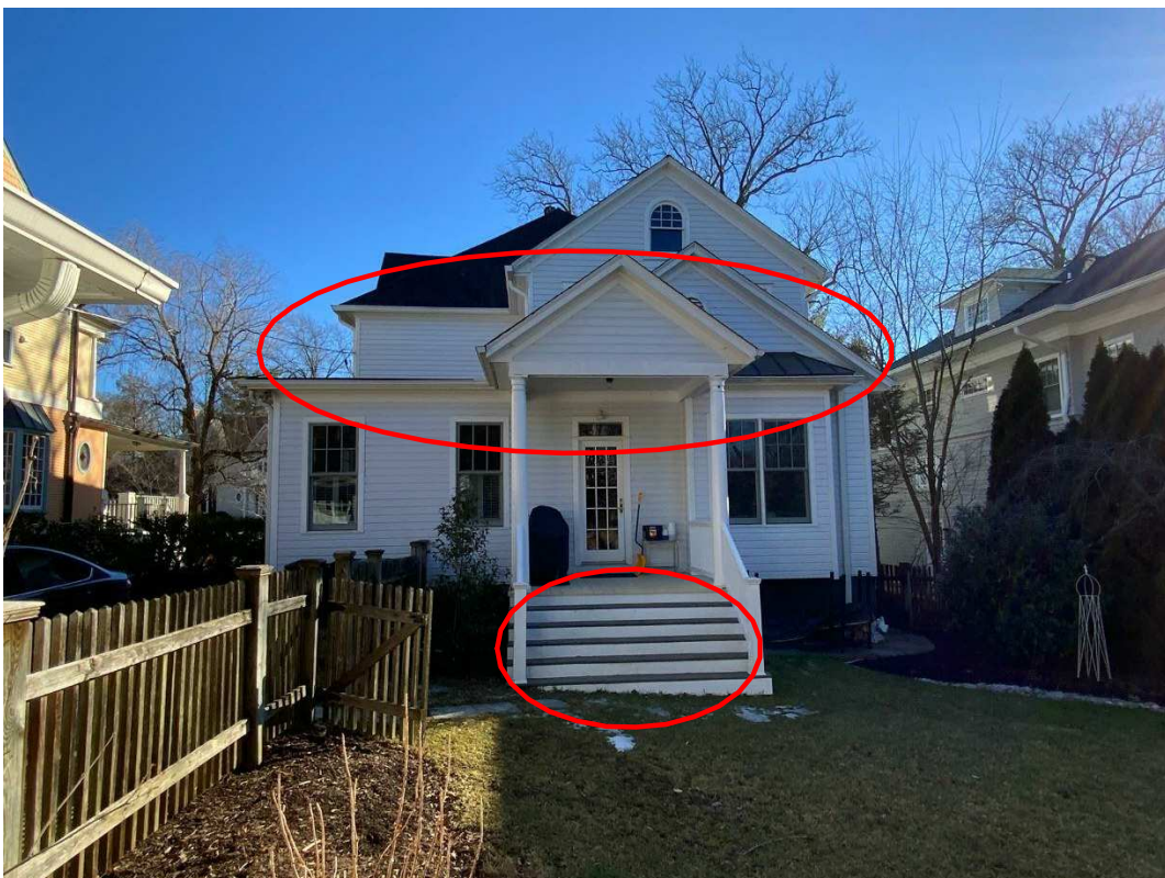
Detail: REAR OF HOUSE - ROOFS AND STAIR TO BE REPLACED ARE CIRCLED IN RED.
