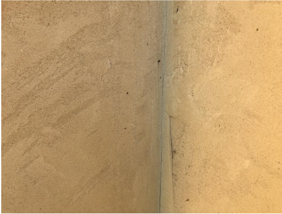
Fig. 3: Chapel building stucco cladding (left) and loggia stucco cladding (right).
