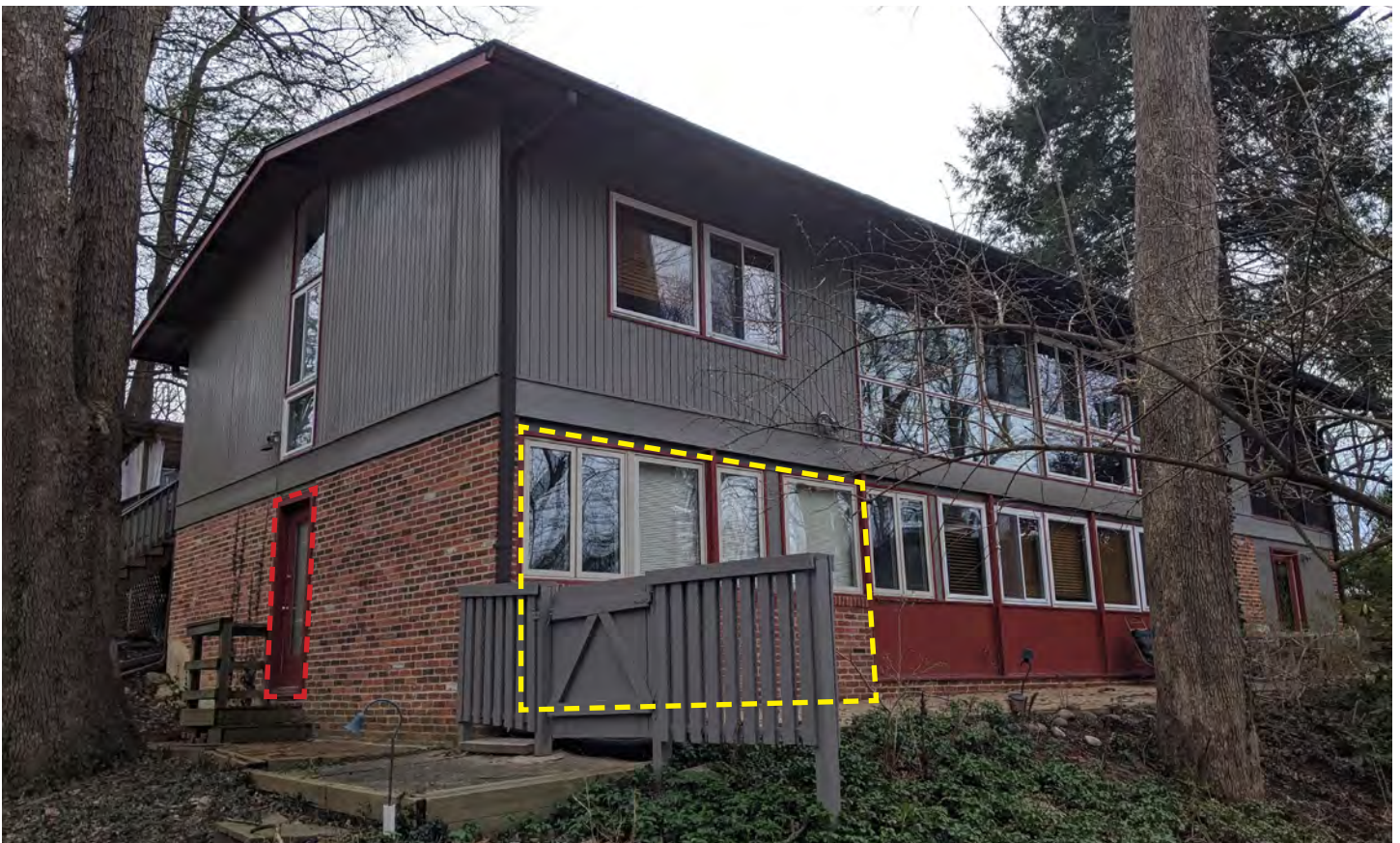
View of the west and north elevations. Alterations include the infill of the first-story recessed patio and entry (dashed yellow line) and potential installation of a single-leaf door (dashed red line).
