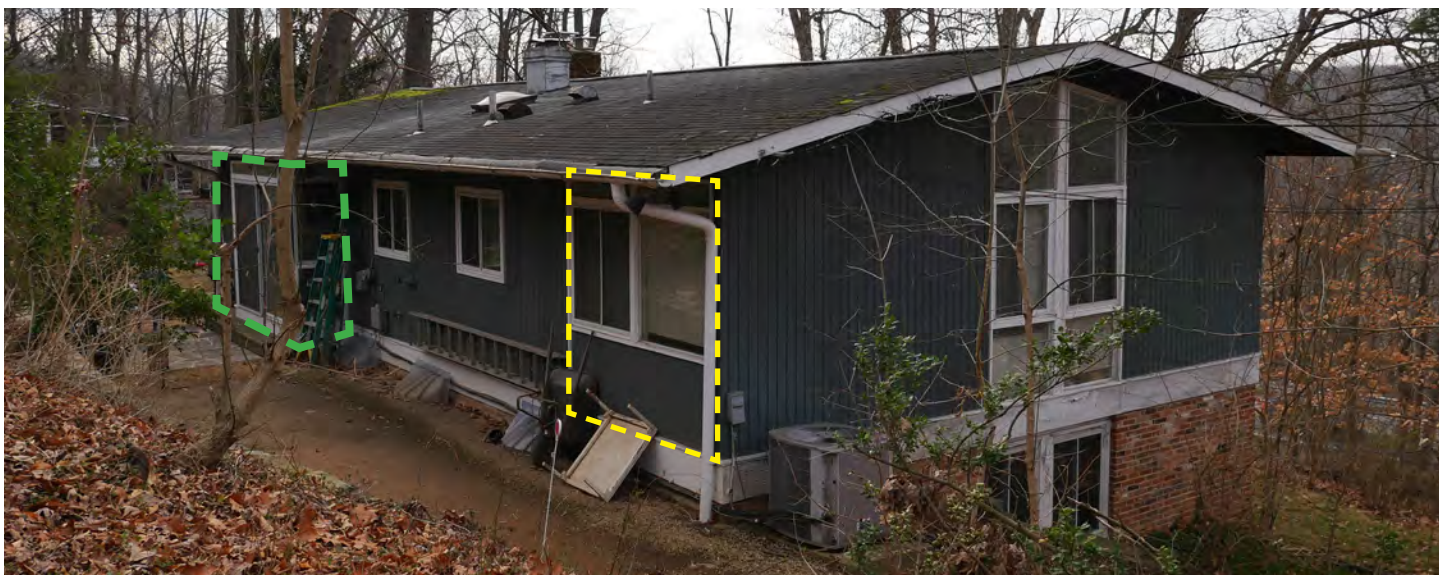
View of the east and north elevations. Alterations include the construction of a small square bay addition (green box) and potential infill/reconfiguration of the windows (yellow box).
