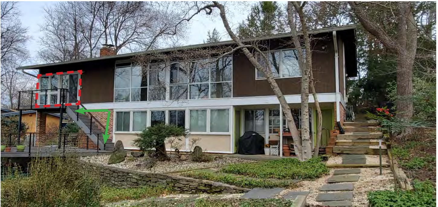
View of the south elevation. Alterations include: 1) the potential enclosure of a screened-in porch and change to the fenestration pattern (dashed red line); and 2) construction of a multiple-level balcony and deck on the southwest corner of the building (green arrows). The balcony and deck were built in 2009.
