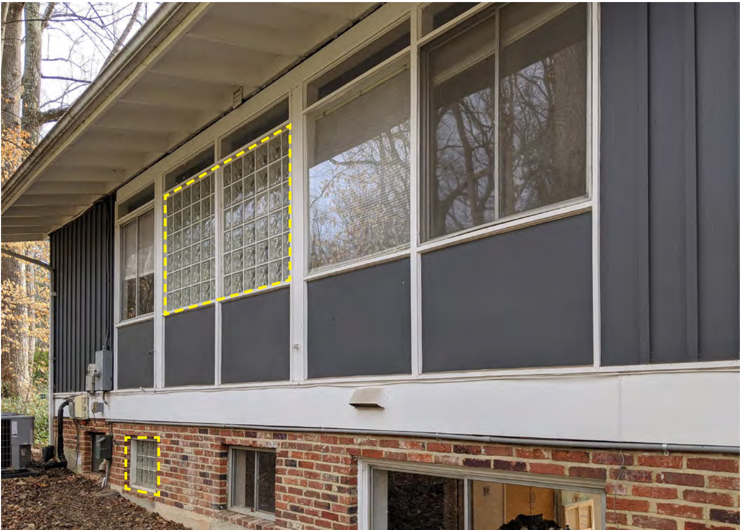
Detailed view of the north (rear) elevation. Alterations include the replacement of the windows with glass block. The size of the window openings, however, remains intact.
