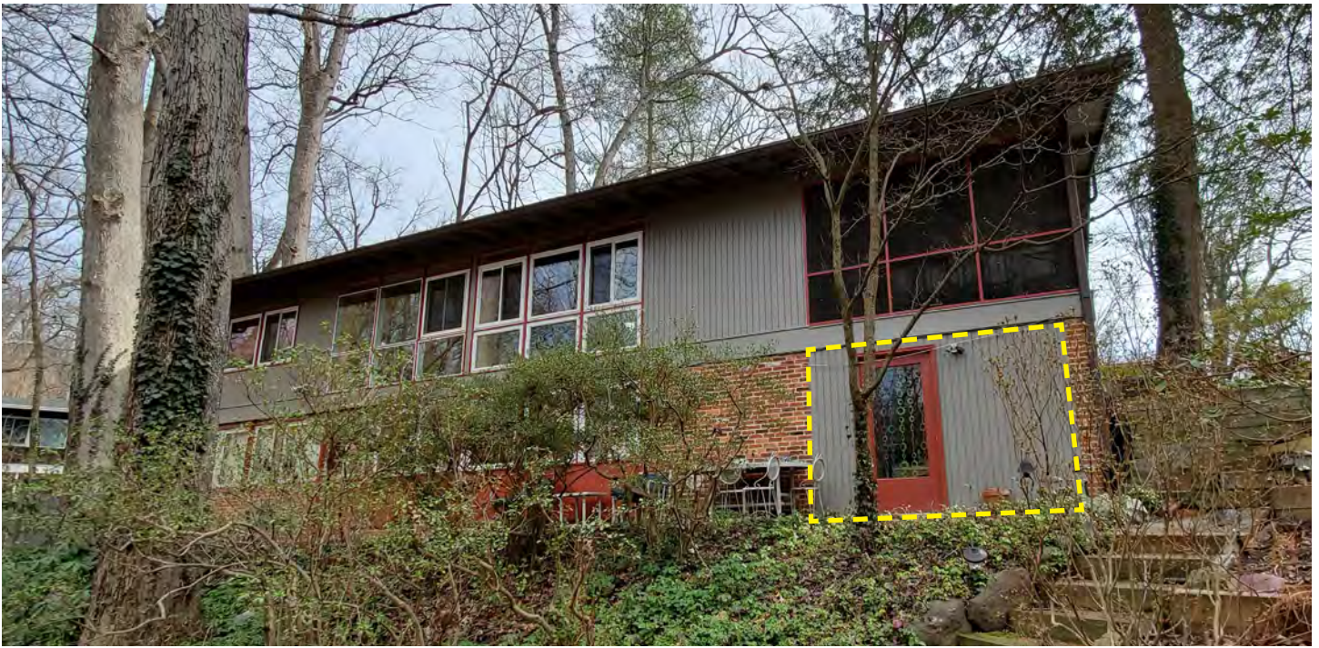
View of the west elevation. Alterations include the infill of the first-story patio (dashed yellow line).
