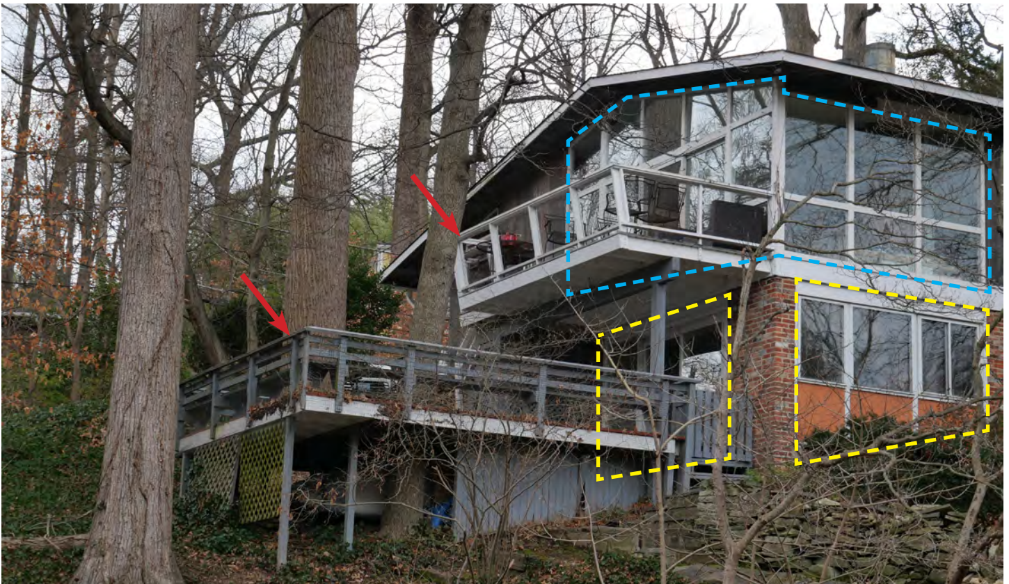
View of the west (rear) and north (side) elevations. Alterations include: 1) the construction of two decks on the north elevation (red arrows); 2) infill of an open patio (dashed yellow line); and 3) enclosure of a screened-in porch (dashed blue line).
