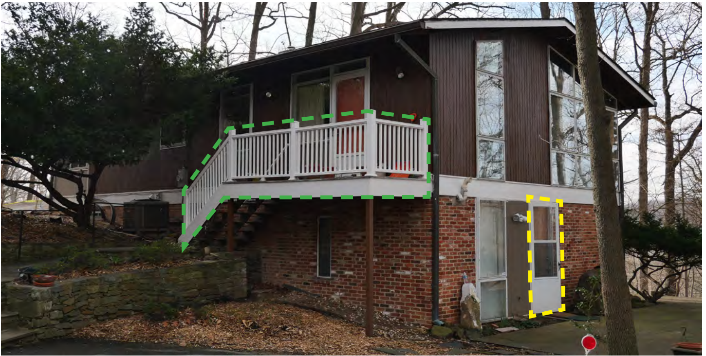
View of the north and east elevations. The first story consists of numerous alterations including the addition of a single-leaf door (yellow box). No other Highview models have doors on the gable ends. The location of the historic deck and stair (green box) on the west elevation is original, but features a non-historic balustrade.
