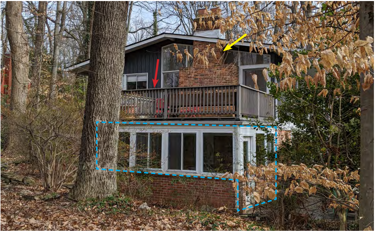
View of the west and south elevations. Alterations include the infill of the patio (dashed blue line) and replacement of the original porch railing (red arrow). The yellow arrow points to the brick chimney stack which is atypical for this model. The other models had a brick base and metal flue.
