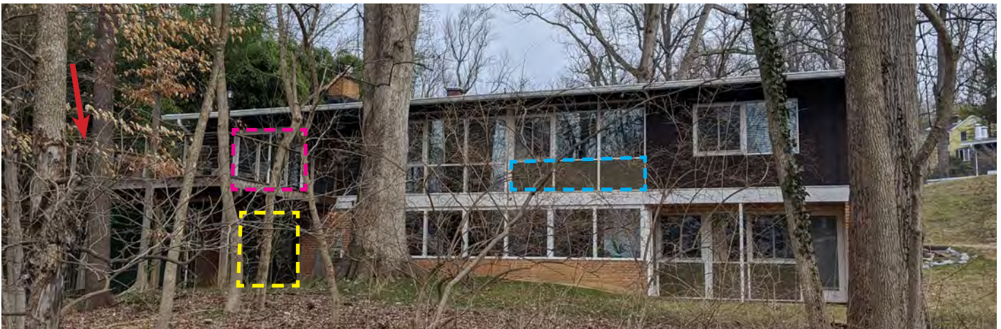
View of the west (rear) elevation. Alterations include: 1) the infill of fixed-light windows with wood panels (blue dashed line); 2) the enclosure of a first-story patio (dashed yellow line); 3) replacement of a window opening with a sliding glass door (pink dashed line); and 4) construction of a deck (red arrow).
