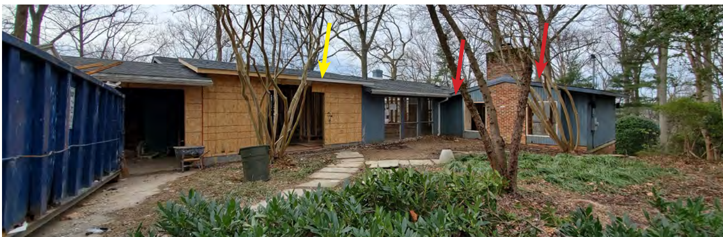
View of the north elevation showing ongoing renovation, 2020. The red arrows points to the infilled breezeway and carport with non-historic brick chimney and fenestration. The yellow arrow points to the current infill of a non-historic breezeway that accessed the current carport for a new primary entry. The addition has a raised shed roof that pierces the slope of the gable roof.
